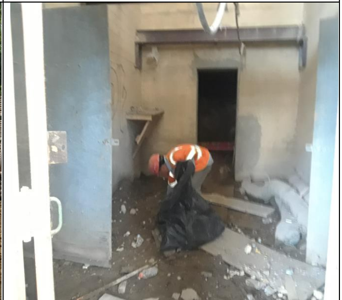
Picture showing cleaning at Roselyn abutment
