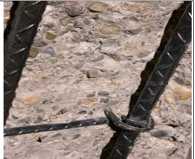
Newly wire brushed patch ready for painting
