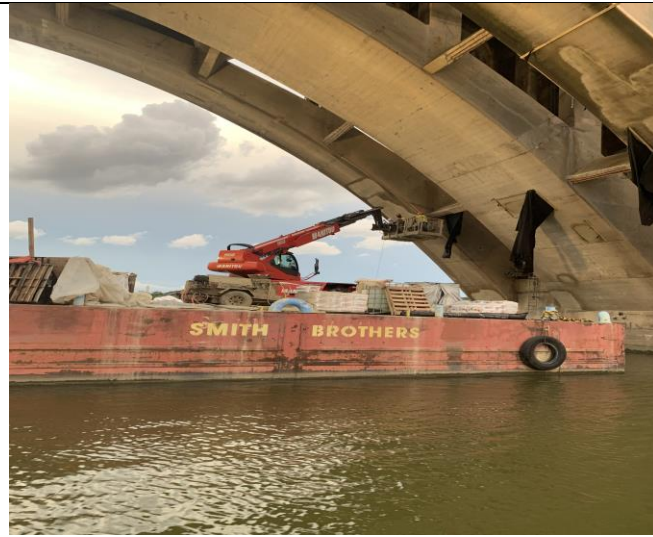
Technopref building containment for demolished marked delaminated concrete at Span H
