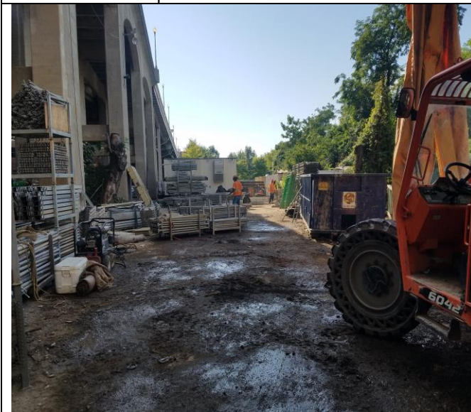
Technopref arranging scaffolding stockpiles & plywood in the staging area for demobilizing
