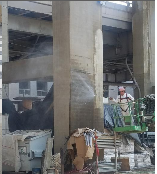
Technopref on East Ramp surfaces power washing post shotcrete surface residue
