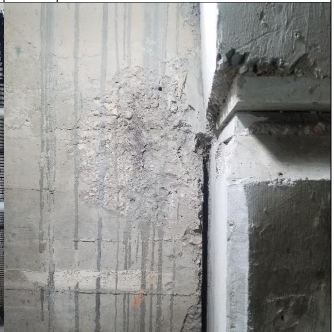
Technopref post strip touch up on Bearing Replacement at N Abut on Row EE, W Elev at Span B
