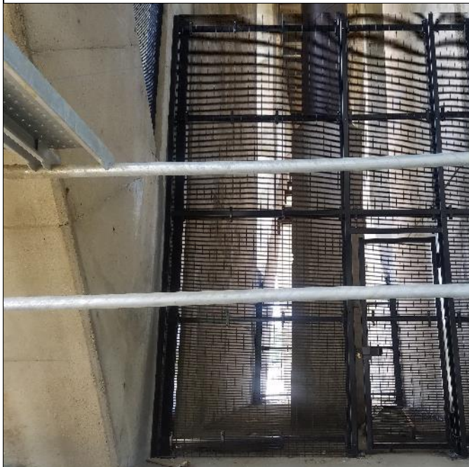
Suburban installed 16' tall Security Fence at South Abutment Bay 2 completed & measured
