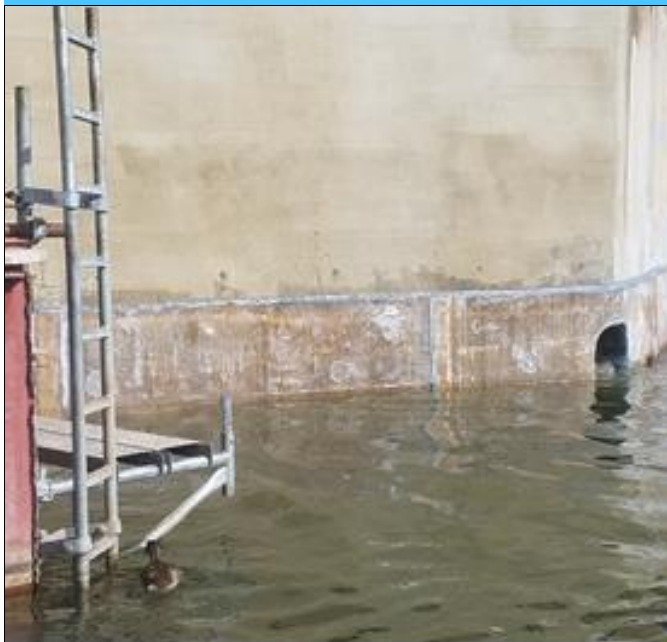
SUS at Pier 1 N & S Elev with Technopref stripping form and prep to inject grout
