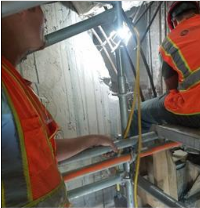
Rebar installation for bearing replacement at North Abutment
