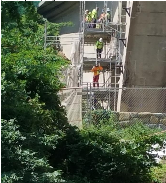
Brock Services at Rosslyn Abut dismantling scaffolding system
