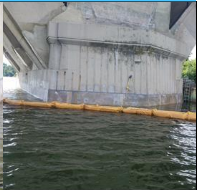
SUS at Pier 1 N Elev with Technopref prep to inject grout - Encapsulation
