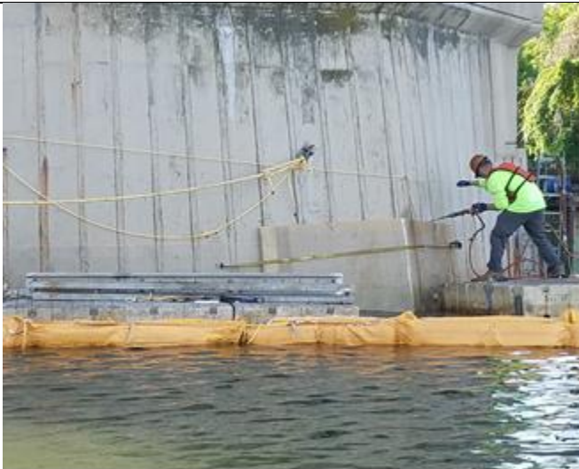
Temporary support for the bearing replacement at the North Abutment.
