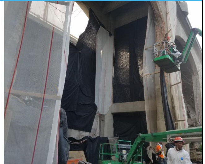
Installing containment at East Ramp for shotcrete operation
