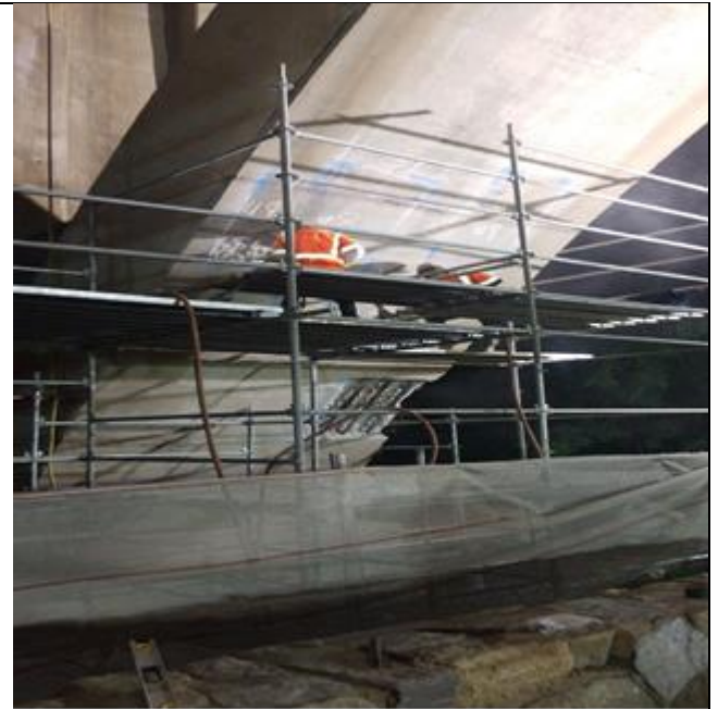
Concrete repair and saw cutting at South Abutment during night shift
