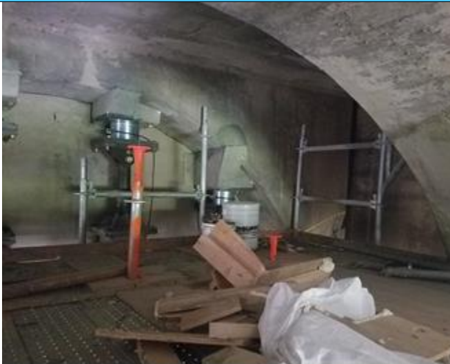
Temporary support for the bearing replacement at the North Abutment.
