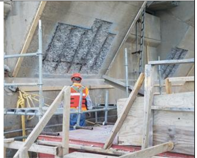
Concrete repair and saw cutting at Pier 2
