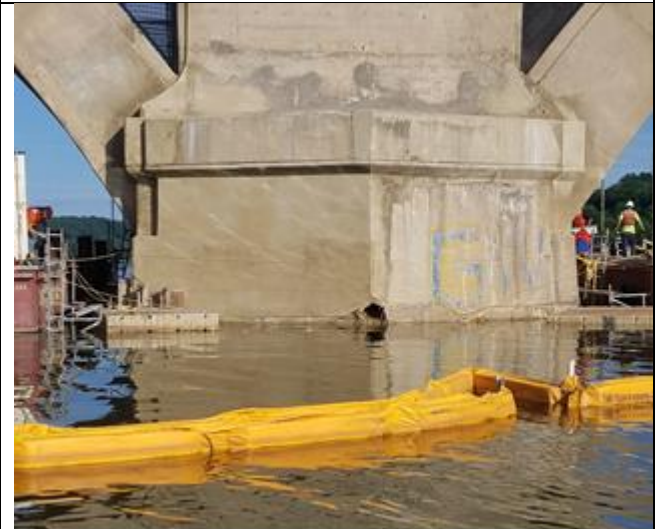
Installing containment at East Ramp for shotcrete operation
