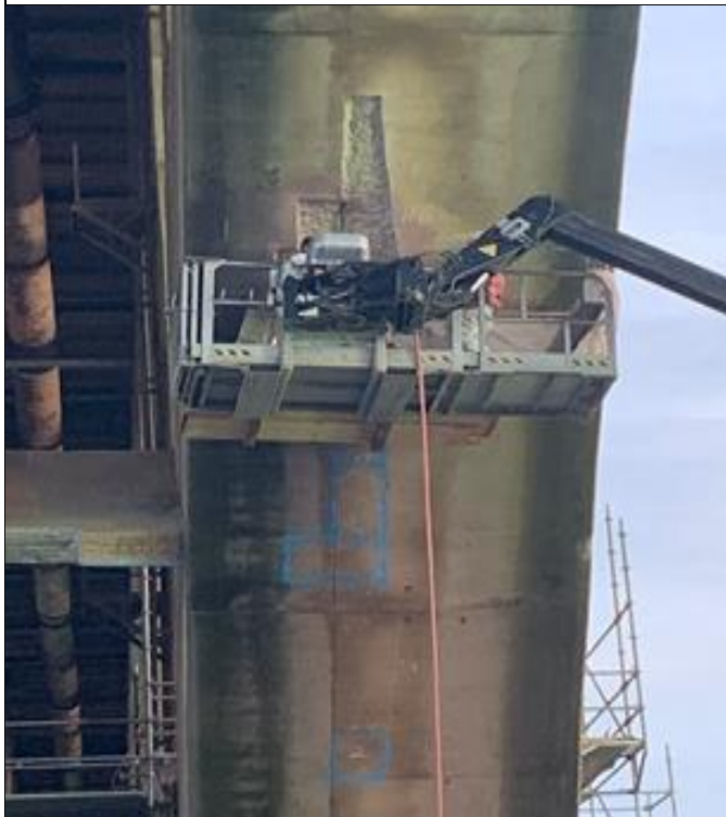
Concrete repair and saw cutting at Span E
