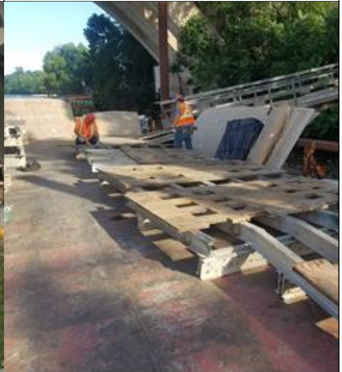
Installing containment at East Ramp
