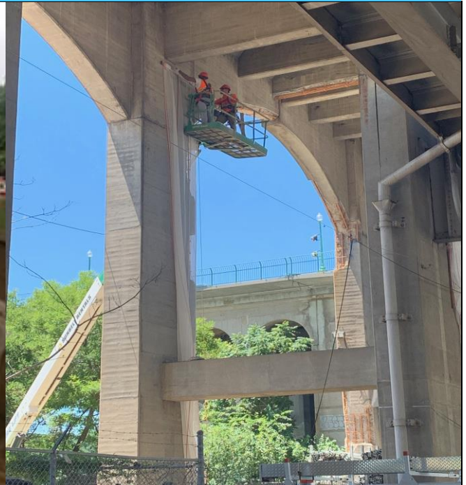
Installing containment at East Ramp
