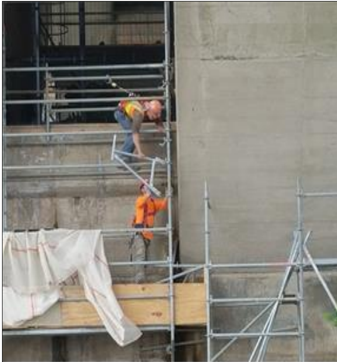
Dismantling scaffold system at South Abutment
