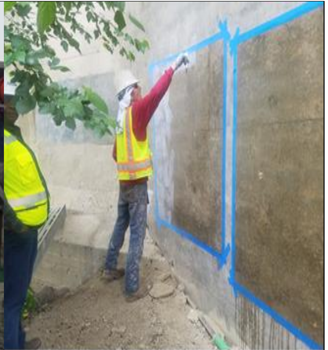
Performing Anti-graffiti application mock up
