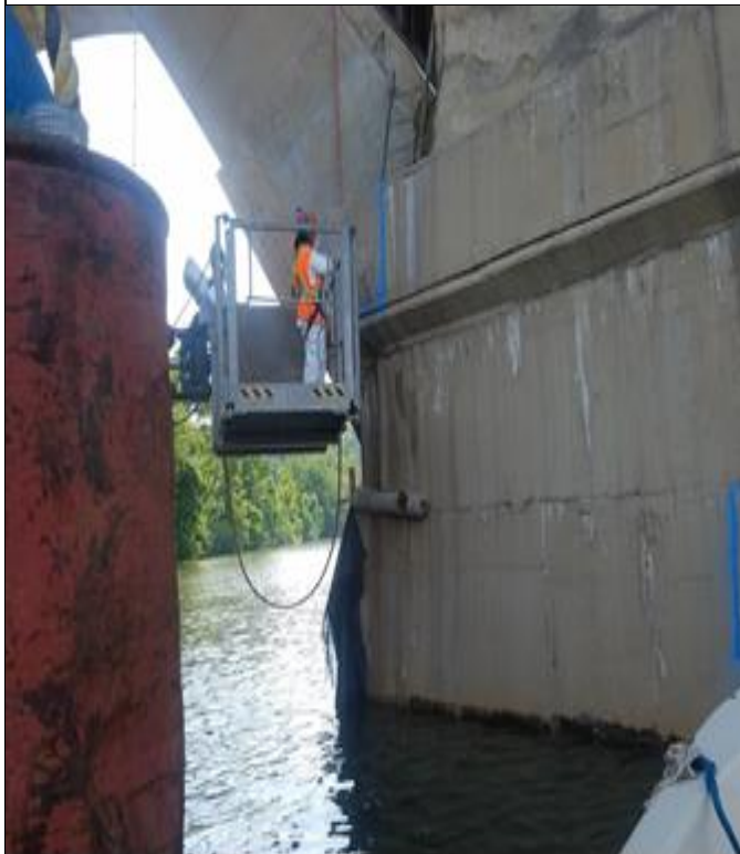
Pier Encapsulation at Pier 2
