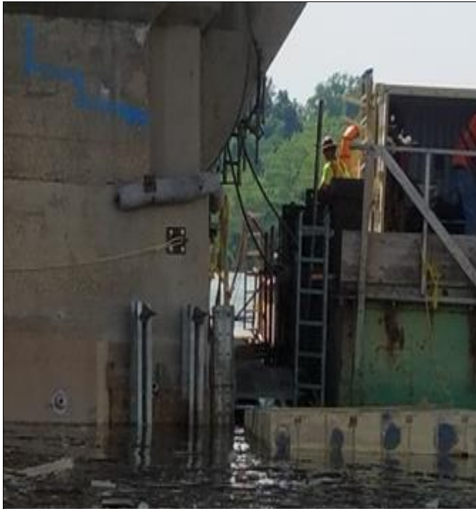
Pier Encapsulation at Pier 2
