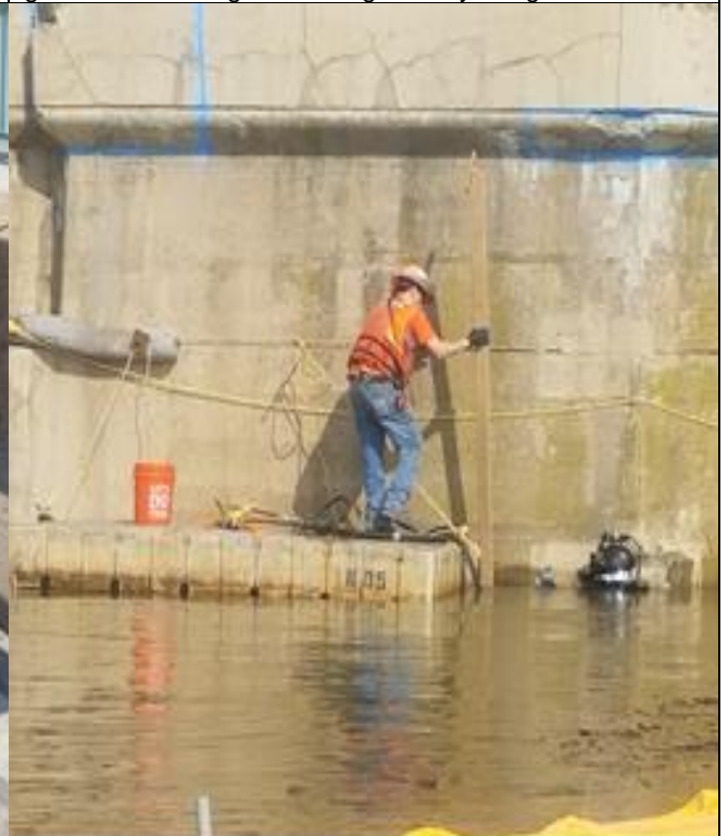
Pier Encapsulation at Pier 2
