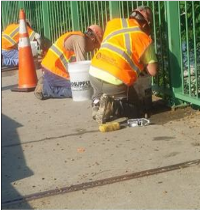
Working on deficiency list for pedestrian railing and placing grout for the railing base along the Key Bridge.
