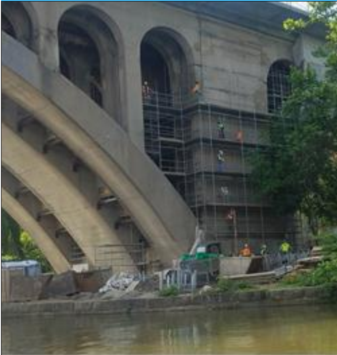
Dismantle scaffold system at South Abutment.
