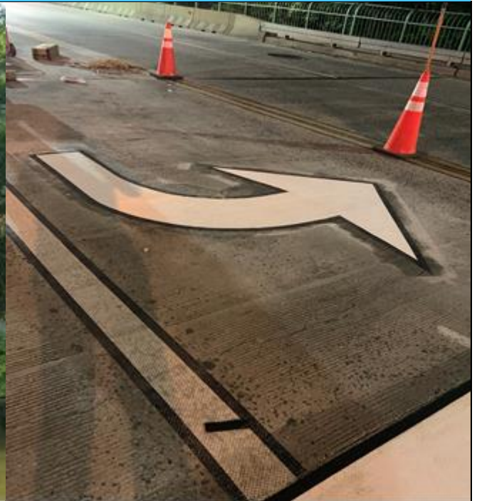
Applying Arrow symbols pavement marking
