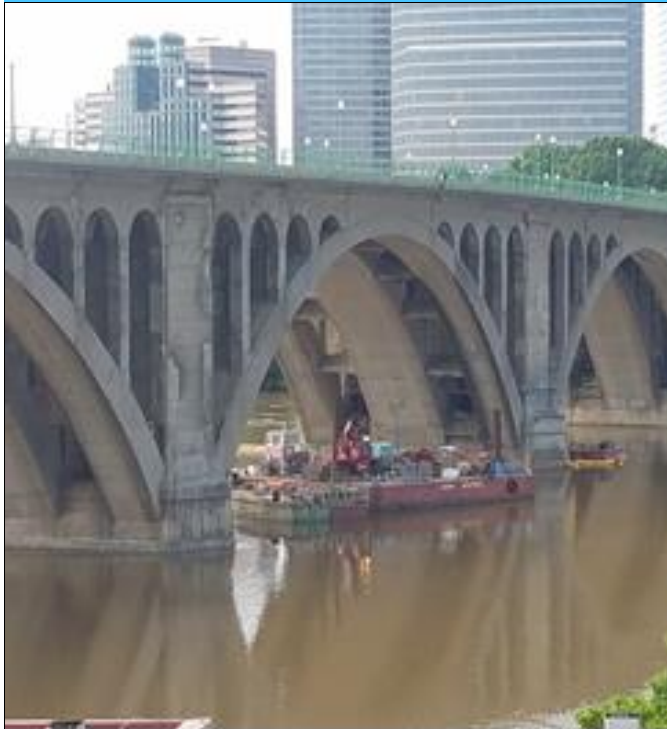
View of of Key Bridge marine operation to repositioning the barges.
