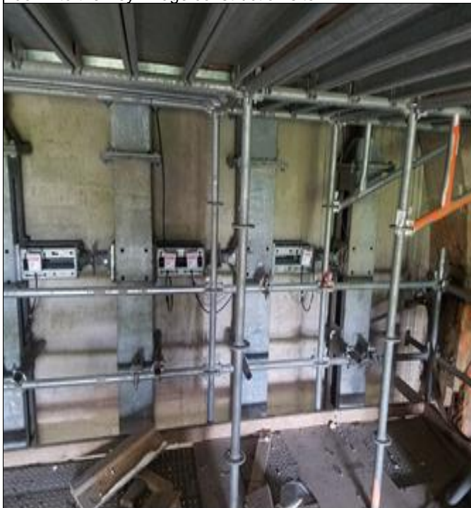
Temporary Support for Bearing Replacement at North Abutment on Row EE
