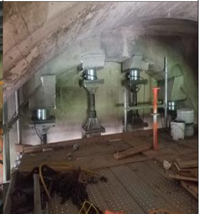
Temporary Support for Bearing Replacement at North Abutment on Row EE
