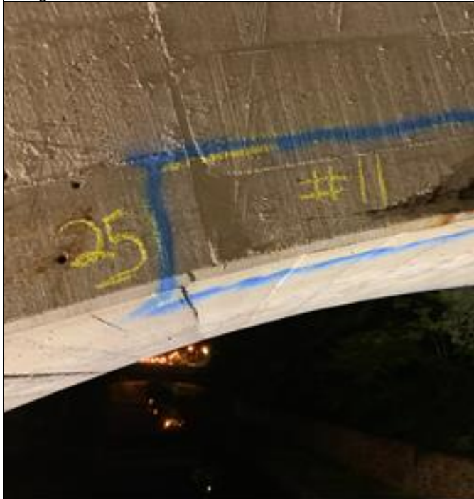
Sounding and marking at Span A
