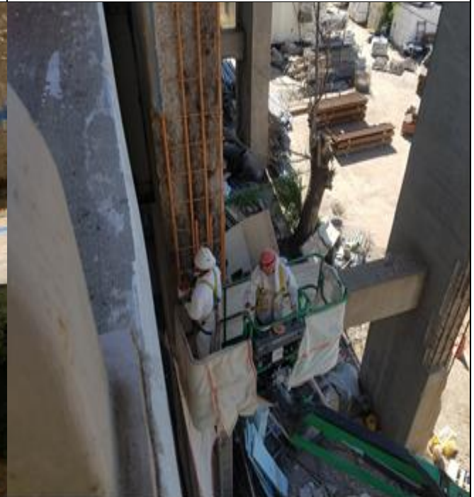
Concrete repair at East ramp by the use of manlift
