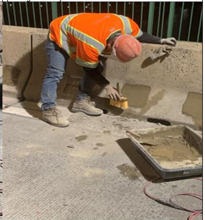
Night work - Working on traffic barrier grout placement
