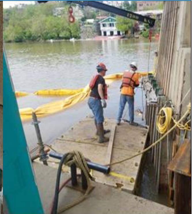
Pier Encapsulation at Pier 3
