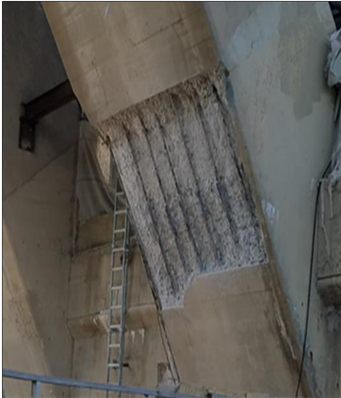
Concrete repairs and demo at Pier 1
