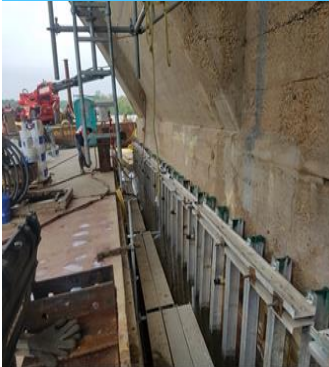
Pier Encapsulation at Pier 3
