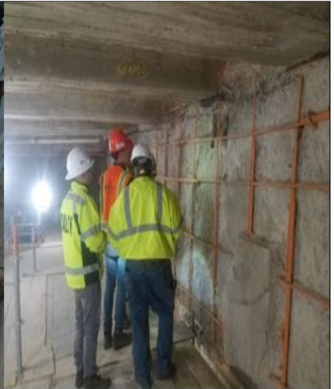
CM & Technopref visit to Rosslyn Approach inspect underpinning & Gallery Floor Slab concerns
