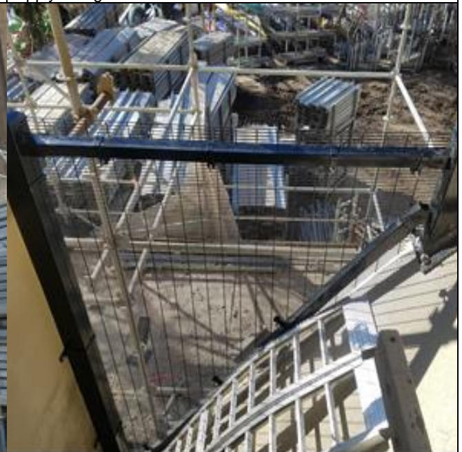
Subcontractor at N Abut started installation of Security Fence
