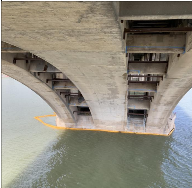
Span E Diaphragm beams sounding
