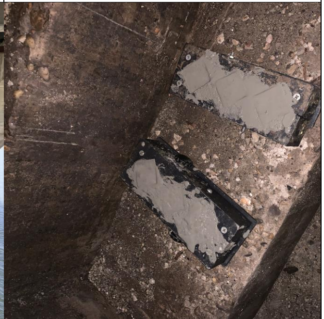
Concrete testing for P5 East chamber deficiency list soffit area
