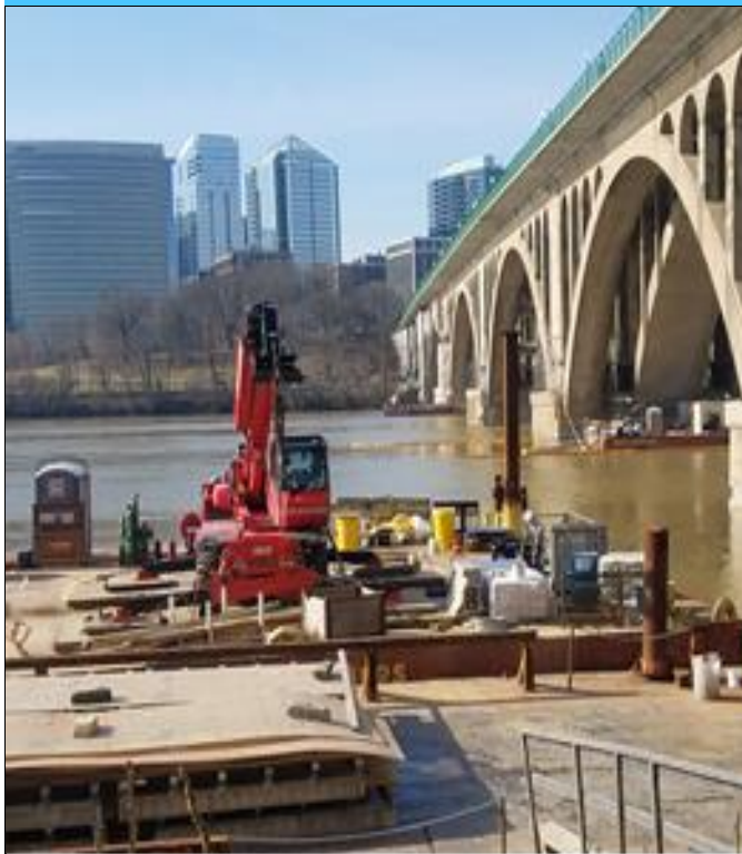
Site Condition from East Elevation view
