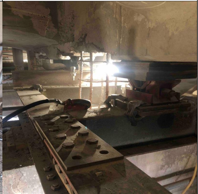
Span G DP 44/45 sandblasted and surf prep approved
