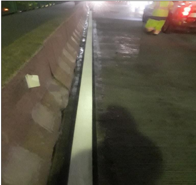
Installed 6" solid white line pavement marking at southbound
