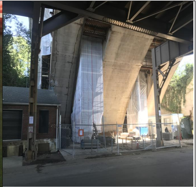
Erection of Scaffolding System at Pier 5
