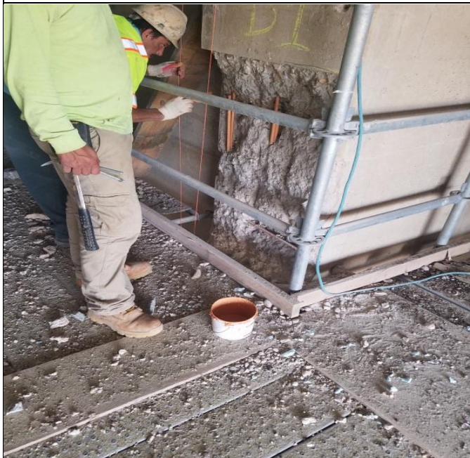
Working on span F FB 51 bay 3 surface preparation.
