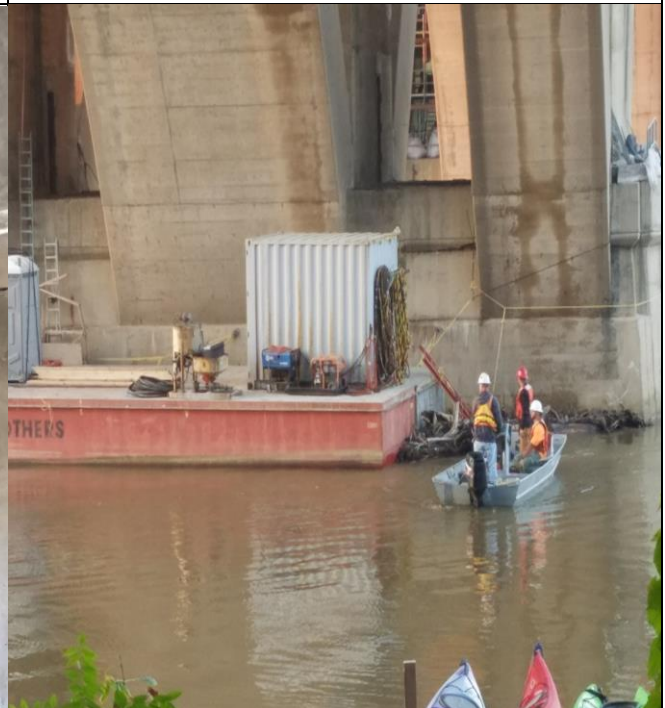
Specialty Underwater Services for Pier Encapsulation - mobilizing at Pier 4
