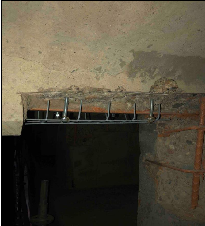
Working on span F FB 51 bay 3 surface preparation.
