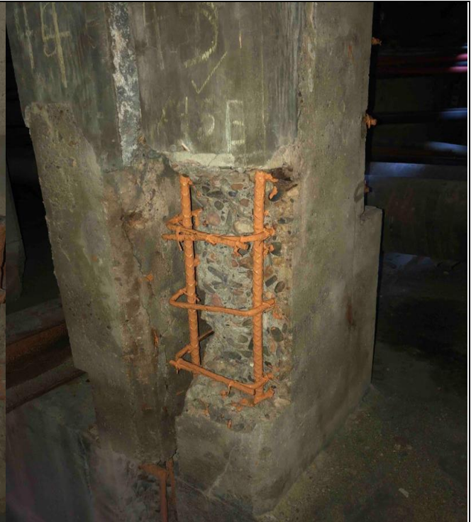
Span G DP 44/45 sandblasted and surf prep approved
