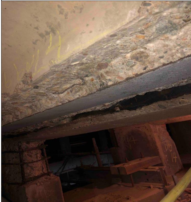
Cleaning rebar on span B DP E11
