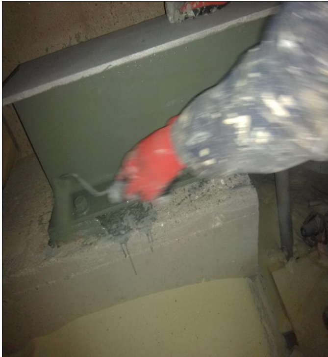
Applying primer paint for Water Main steel supporting beam
