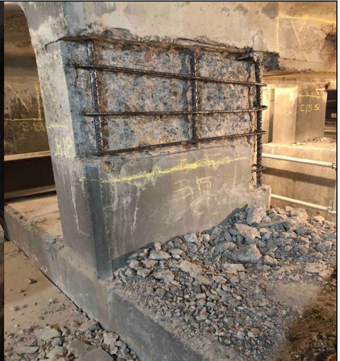
Span B B15 demo and surface prep approved
