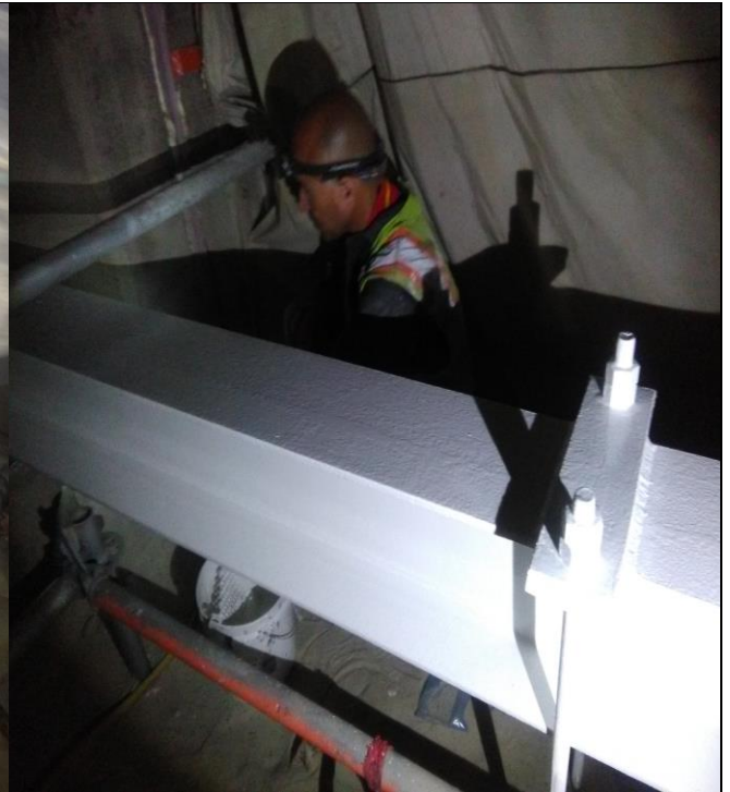
Applying intermediate paint for Water Main support beams in span E
