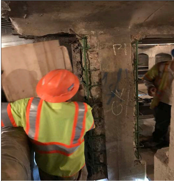
Installing formwork at Span C deck pedestal A34
