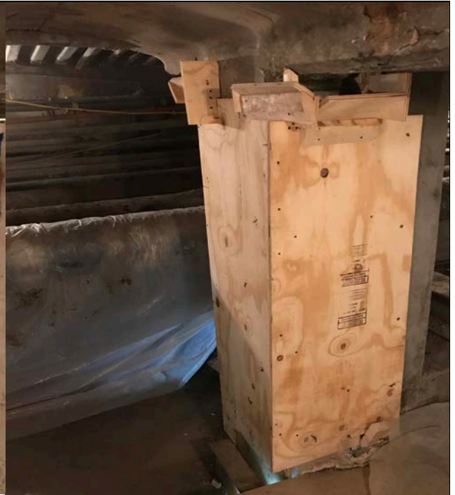
Finished formwork at Span C deck pedestal A34
