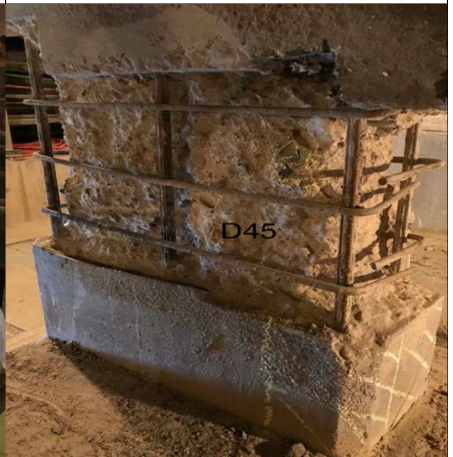
Inspection of Span D deck pedestal D45 concrete demo
