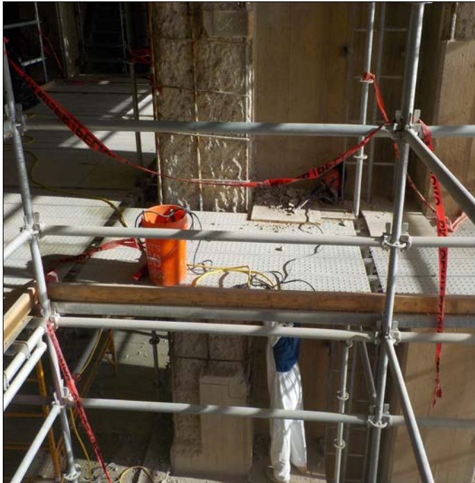
Concrete saw-cutting and chipping at Span E
