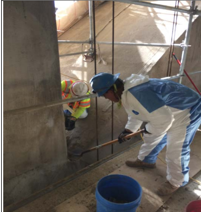
Concrete saw-cutting and chipping at Span E
