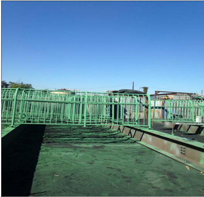
Applying finish coat for pedestrian railing
