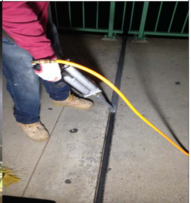
Cleaning and clearing of the dust and debris at non-armored bridge deck expansion joint seals.
