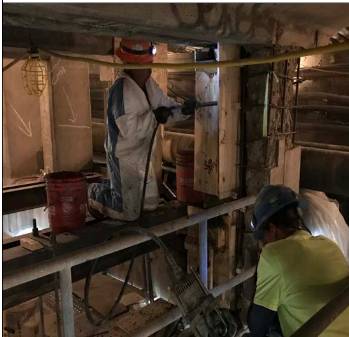
Pouring and vibrating concrete at Span C deck pedestal A25
