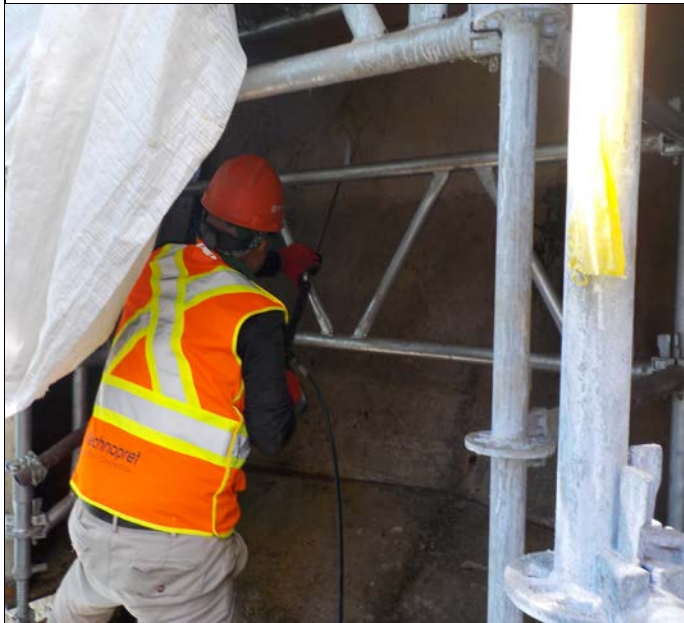
Saw-cutting and chipping at Span D
