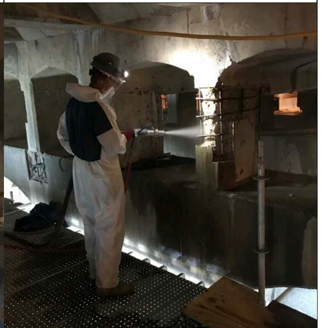
Cleaning Span D deck pedestal D54 with water
