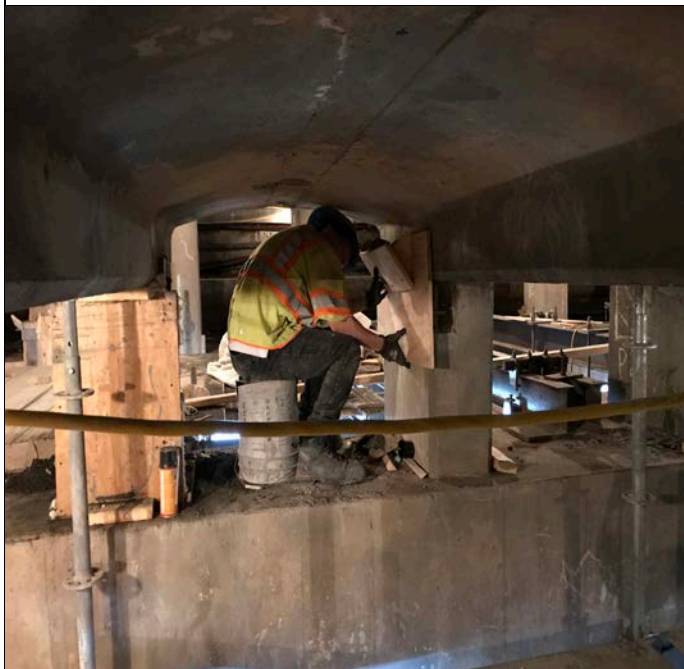
Installing formwork at Span C deck pedestal
