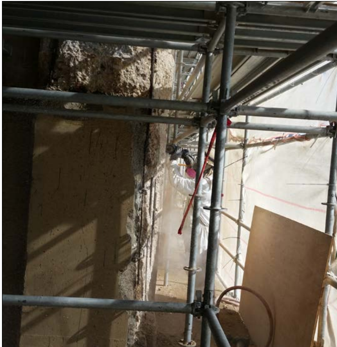
Saw-cutting and chipping at Span D
