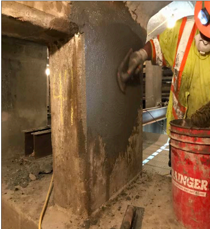
Finishing a Span C deck pedestal with Sika 123
