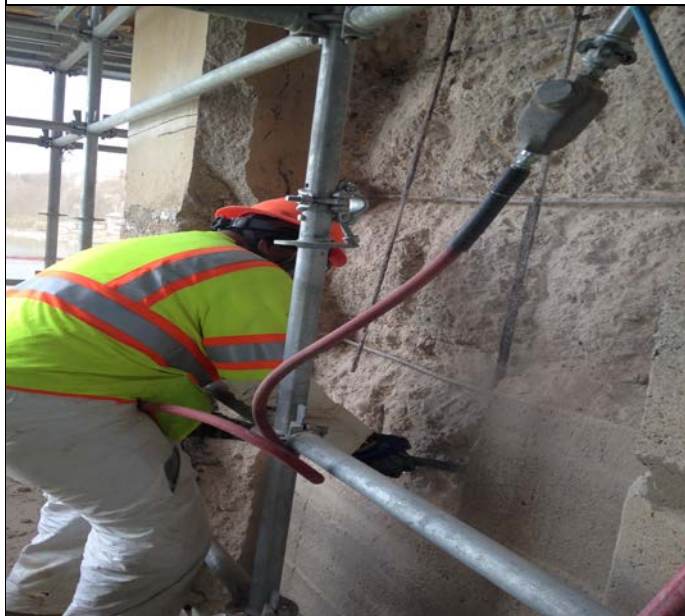
Concrete demoliting at pier 4
