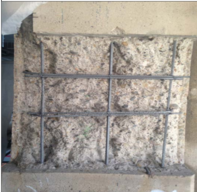
Concrete sandblasting at North abutment
