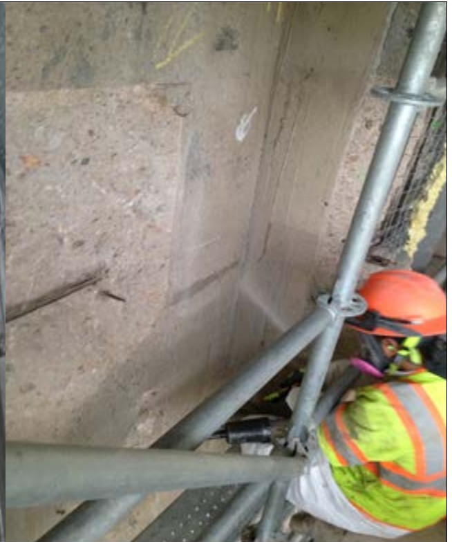
Concrete demolition operation at pier 4
