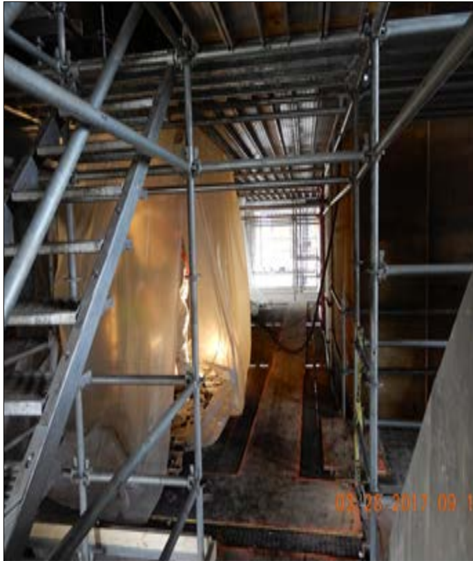
Concrete sounding at pier 4
