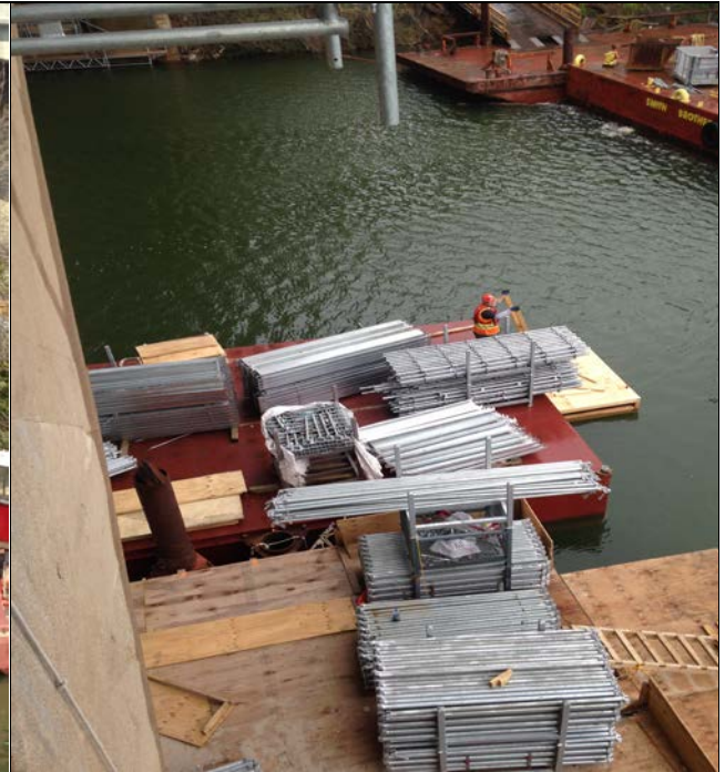
Loading scaffold on barges
