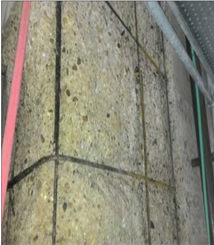
Sand blast area of concrete repair at North abutment
