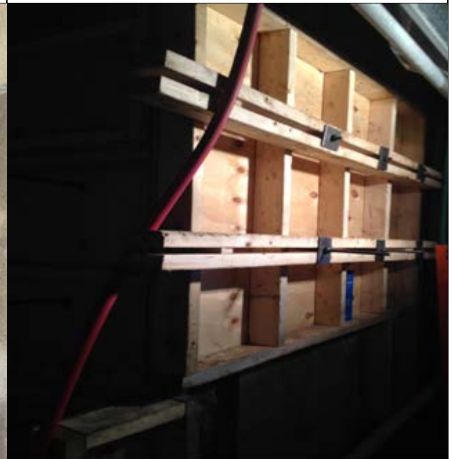
Setting up forms for concrete repair at North abutment
