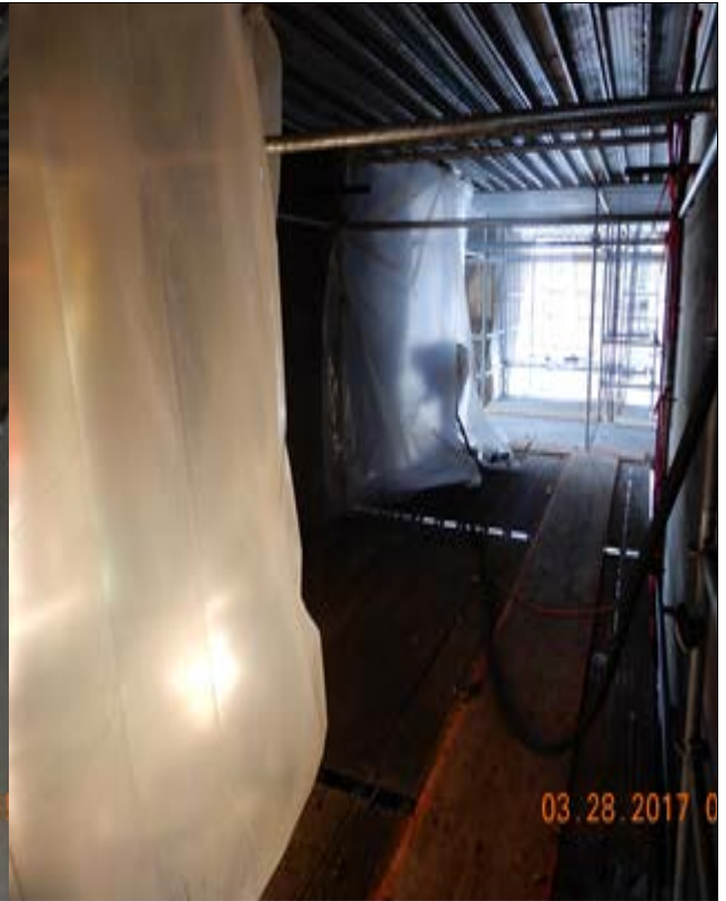
Sandblasting contamination setup for concrete repair
