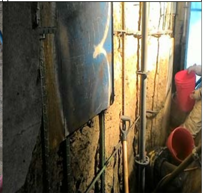
Sand blast area of concrete repair at North abutment
