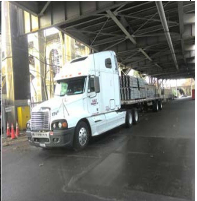
Receiving loads of scaffold
