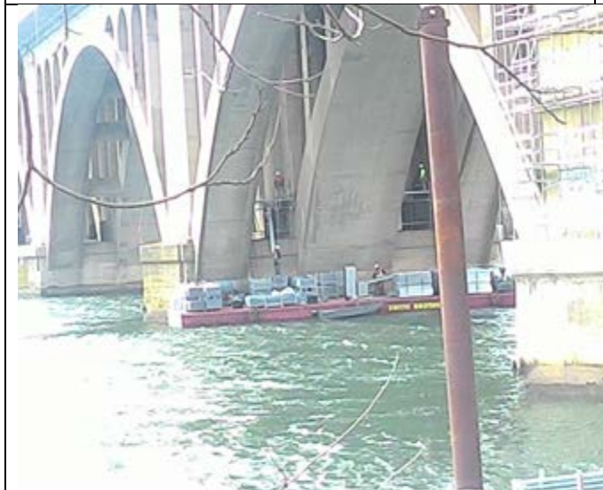
Scaffold instaling at pier 3
