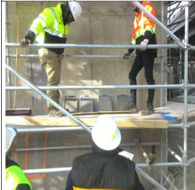
Inspecting samples for matching existing bridge's texture and color
