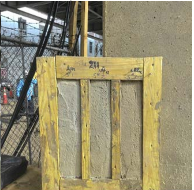
Inspecting samples for matching existing bridge's texture and color
