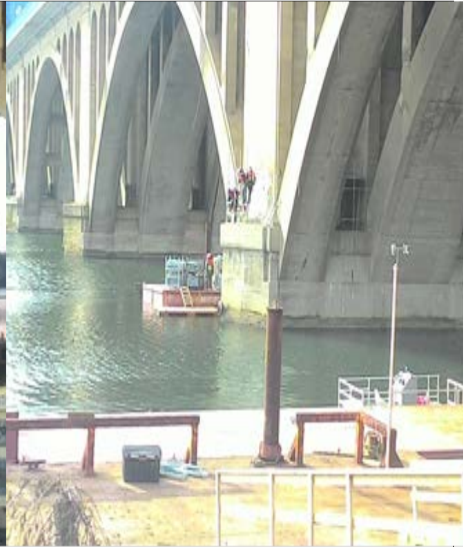
Erecting of scaffold system on pier 4
