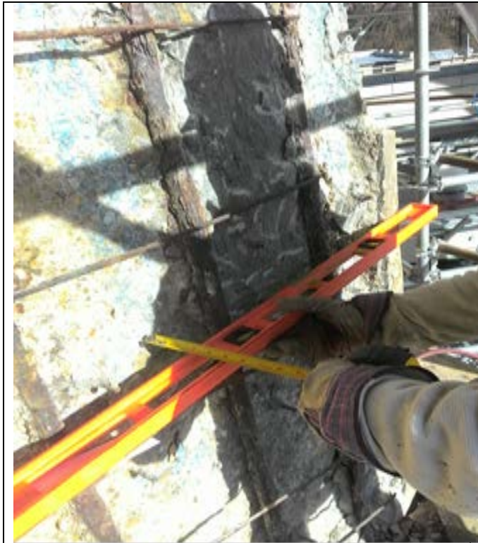
Demo of concrete on N Abut eastside levels
