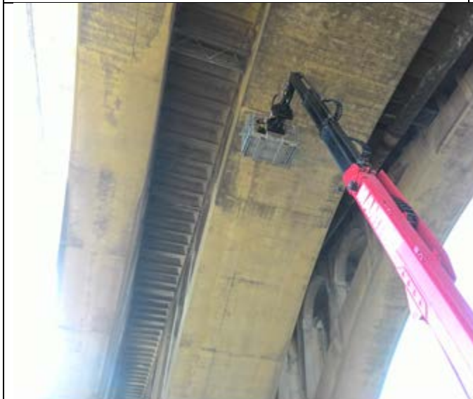
Sounding for span C arch
