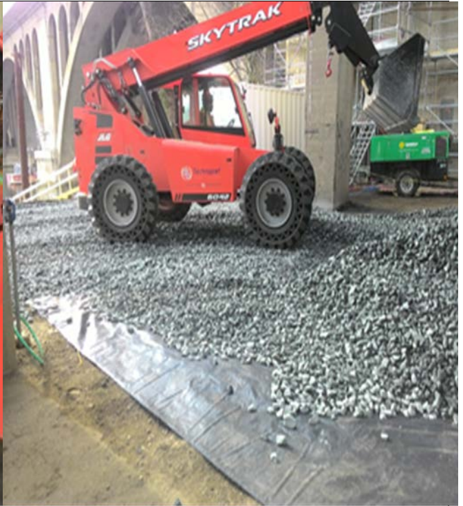
Grading, installing fabric and rip-rap @ the entrance to water access ramp
