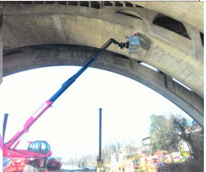
Sounding for Span C arch
