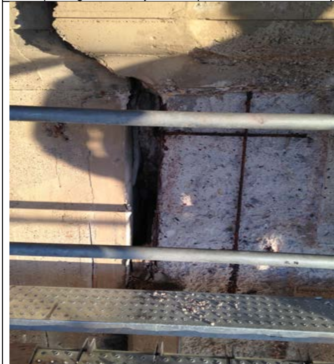
Concrete demo on North abutment westside (unfinished work)
