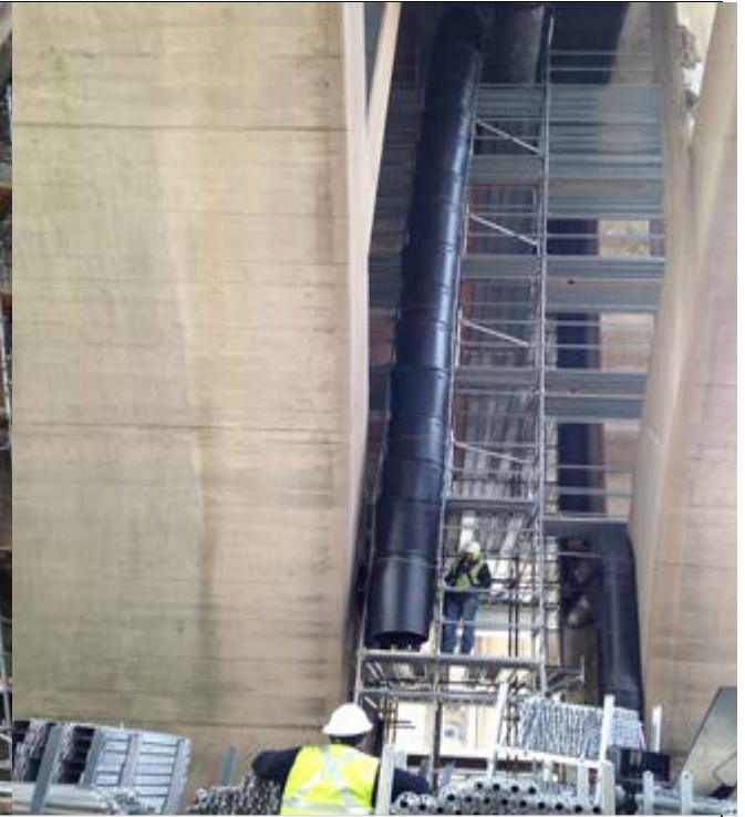
Installation of waste chutes
