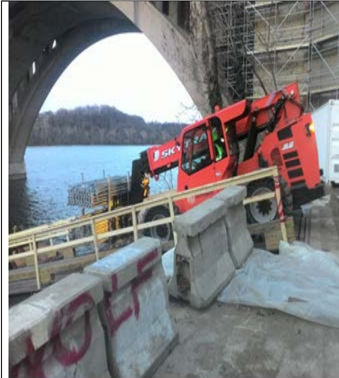
Moving stockpile scaffolding Material onto barges from staging area
