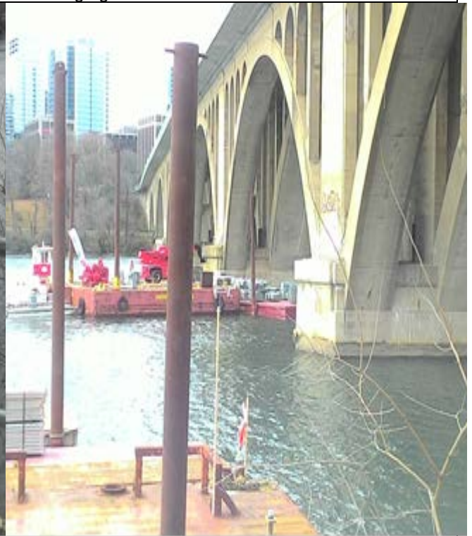
moving Barges to Pier 4 and spudding
