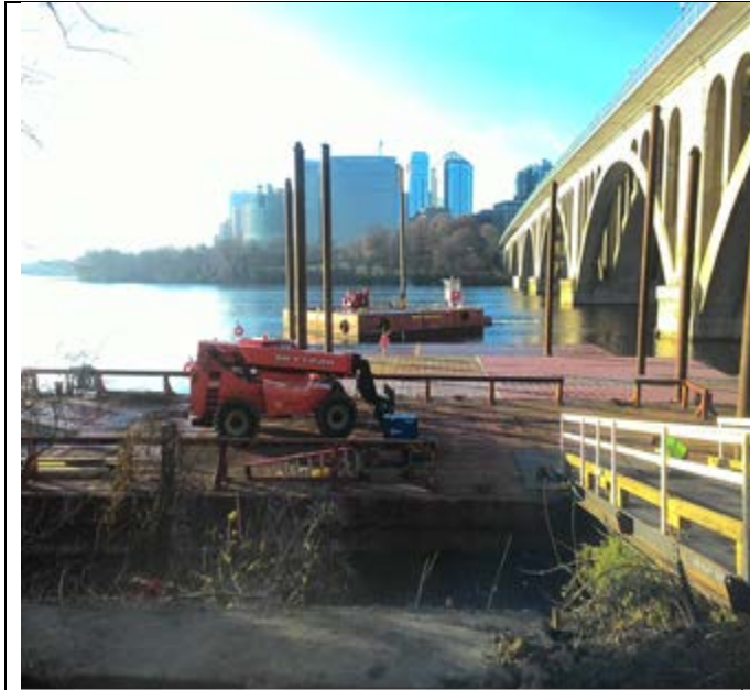
Setting up barges
