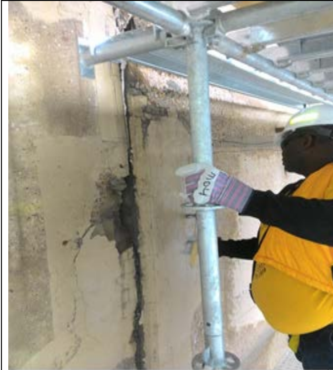
Sounding and layout on North abutment.
