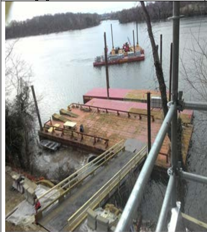
moving Barges to Pier 4 and spudding
