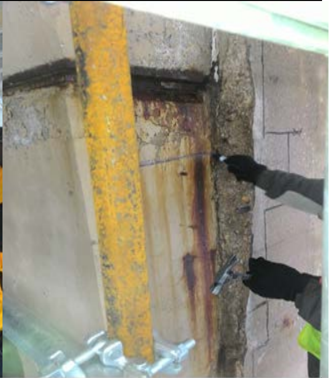
Sounding and layout on North abutment.
