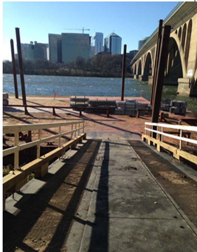
loading barge with scaffolds preparing for pier 4 scaffold installation
