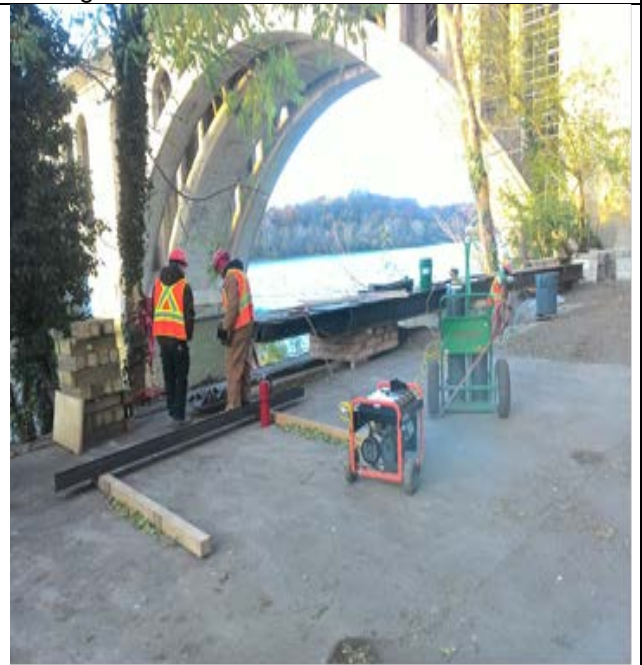
Assembling sections of the water access ramp
