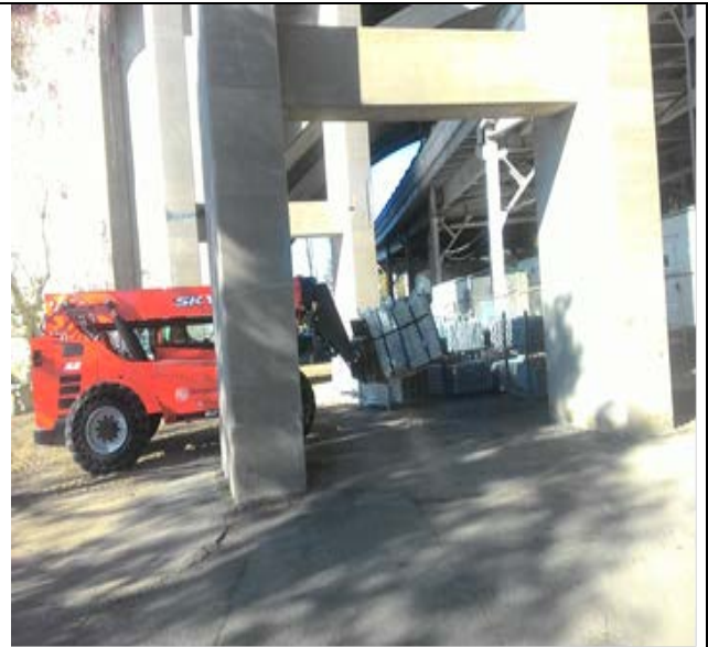
Storing scaffold deliveries
