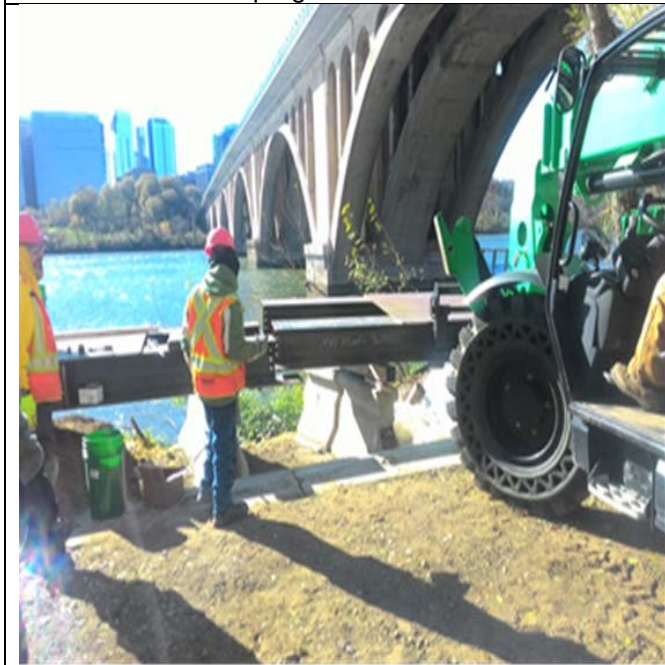
Assembling sections of the water access ramp
