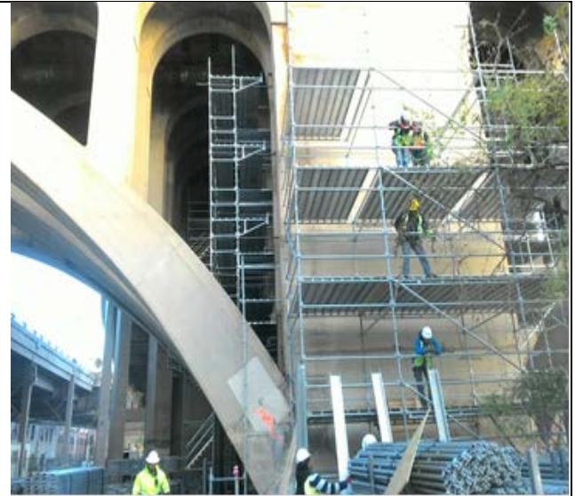
Erection of scaffold progress at North abutment.
