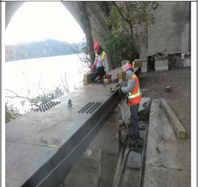
Technopref assembling steel structure ramp for water access
