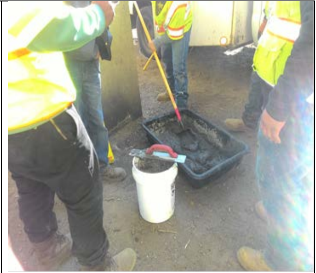
Mixing Pigment and SIKA 123 mixture batch for Coloration Sample
