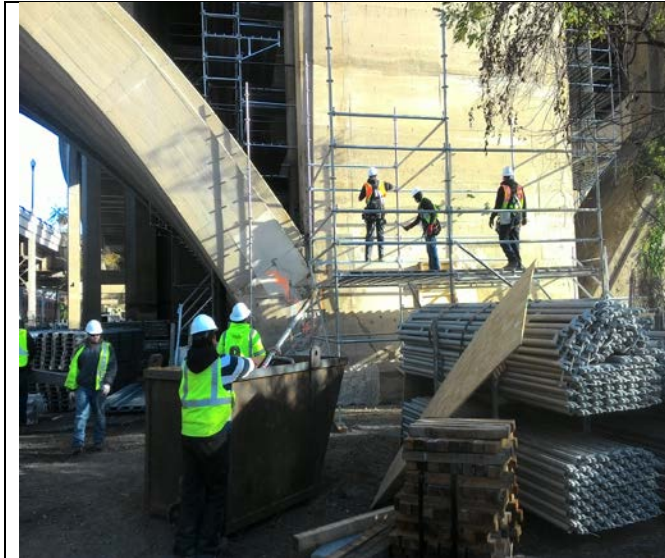
Erection of scaffold progress at North abutment.
