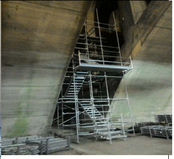
Erection of scaffold progress at North abutment.
