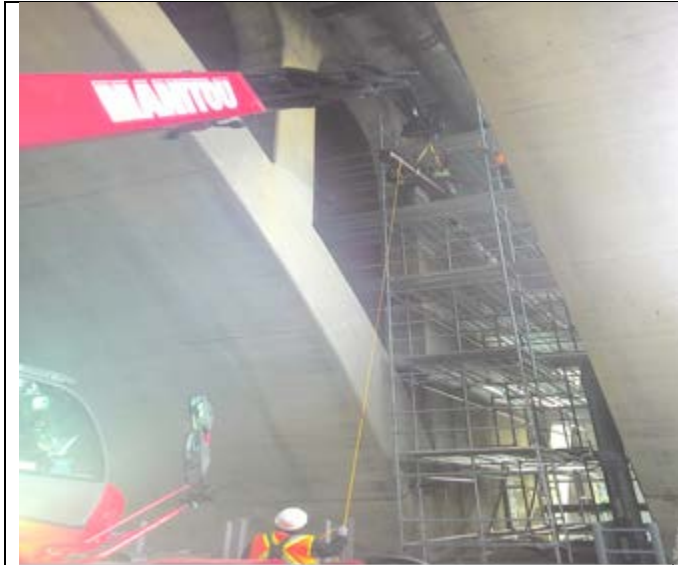
Erection of scaffold progress at North abutment.
