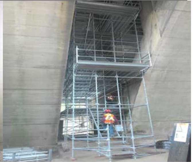
Erection of scaffold progress at North abutment.
