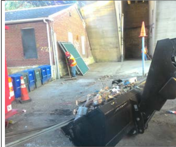
Technopref removed Debris and existing Gate at Pier 5 for Staging Area
