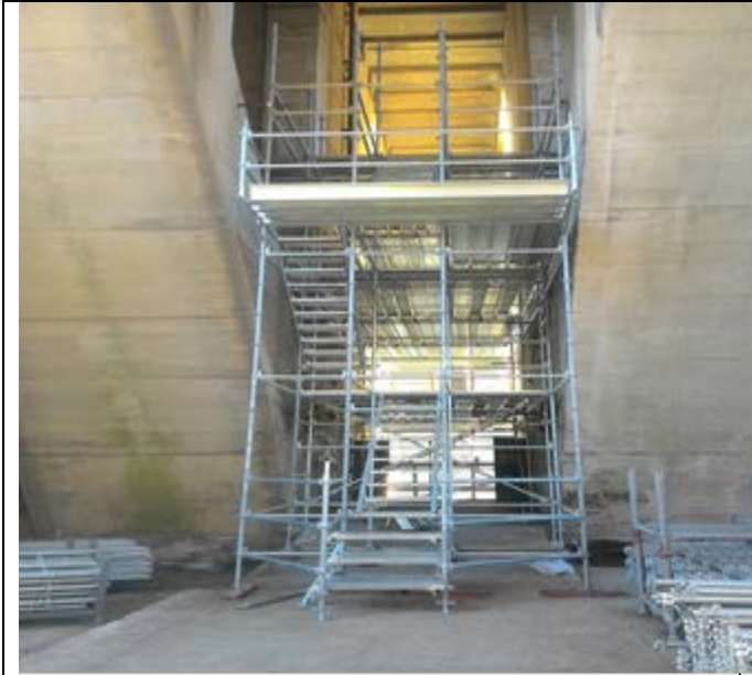
Erection of scaffold progress at North abutment.
