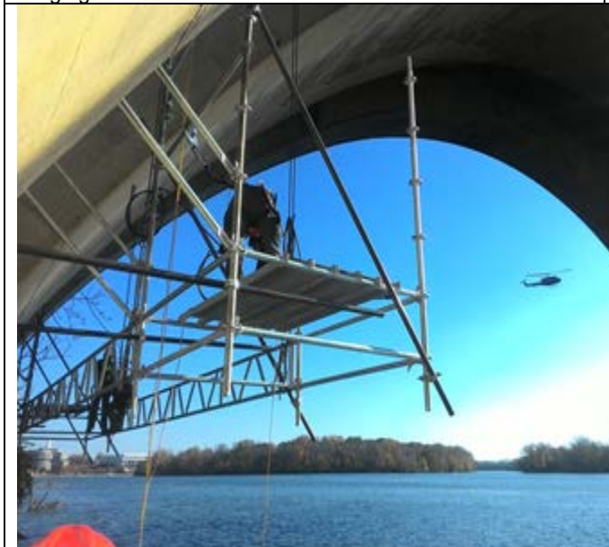
Erection of scaffold progress at North abutment.
