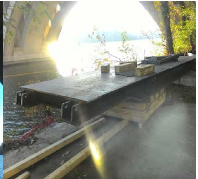
Technopref received steel structure for river access
