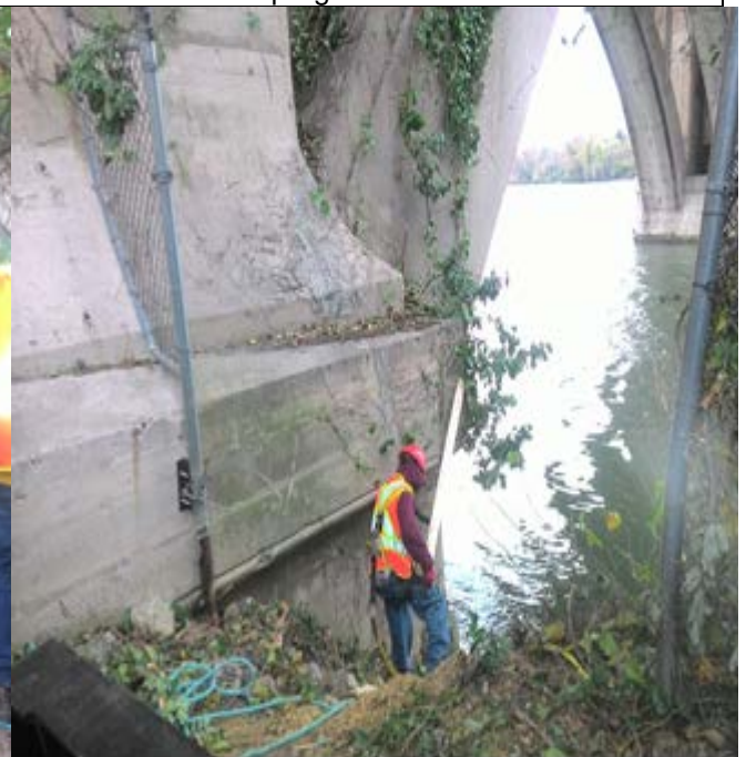
After tree trimming west of North abutment
