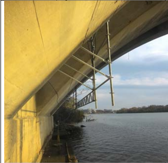
Erection of scaffold progress at North abutment.
