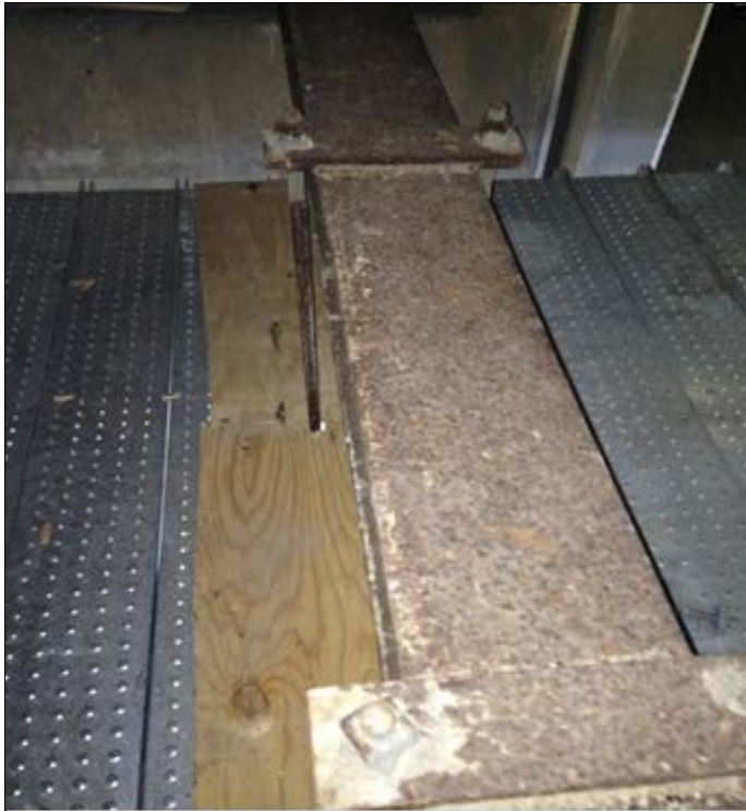
Support beam for Water main before blasting at span C
