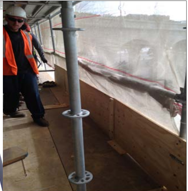
Installation of protection shield at Span D
