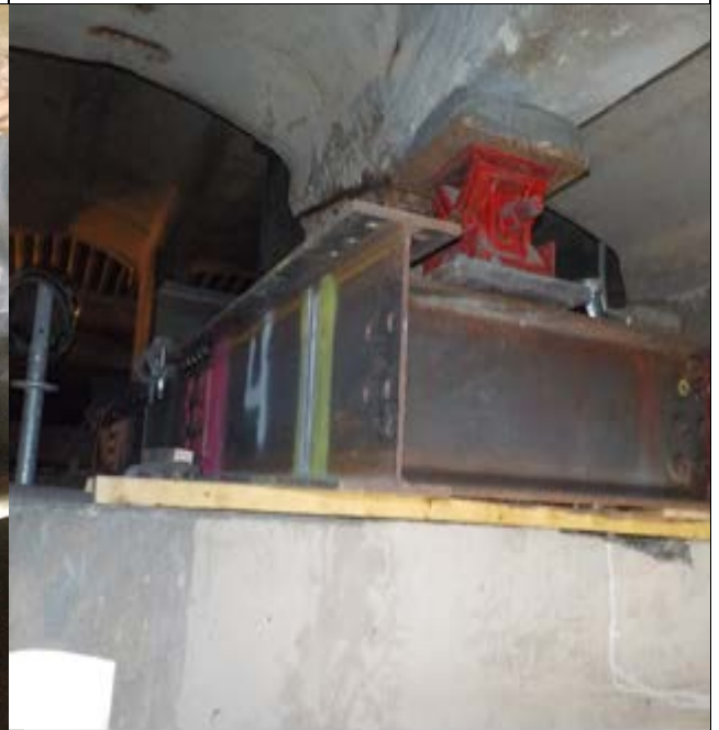
Support beam for Water main after blasting at span C
