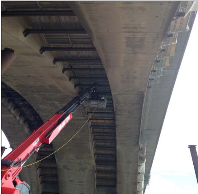
Installation of protection shield at Span D
