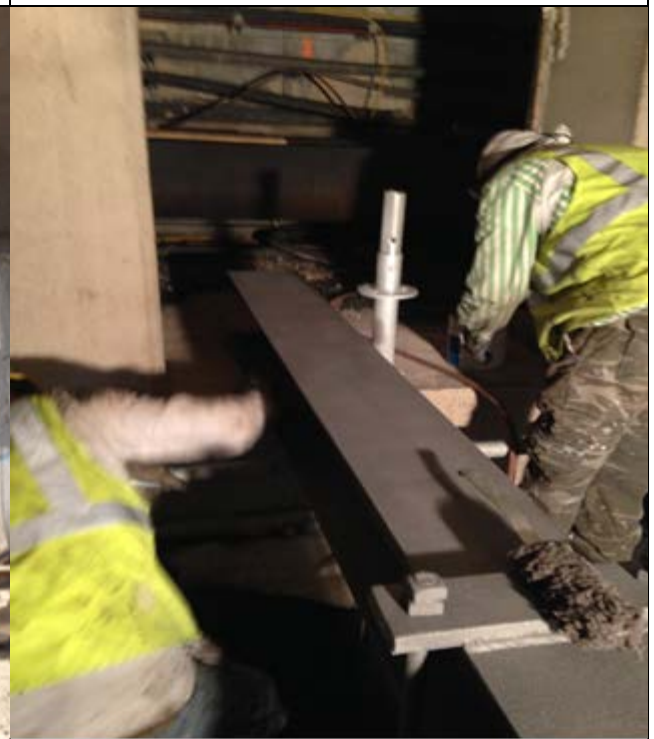
Painting support beam for Water main before blasting at span C
