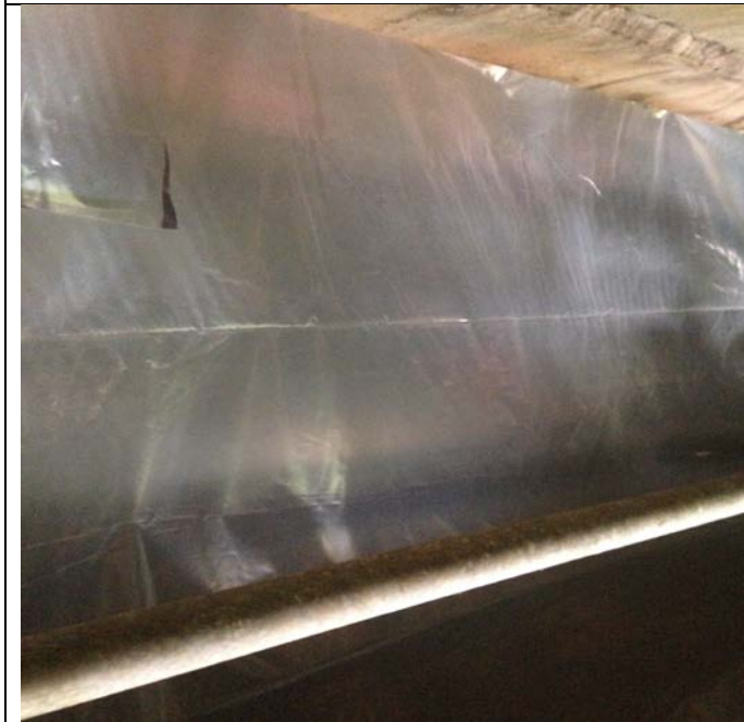
Containment for the water main paint work at span C
