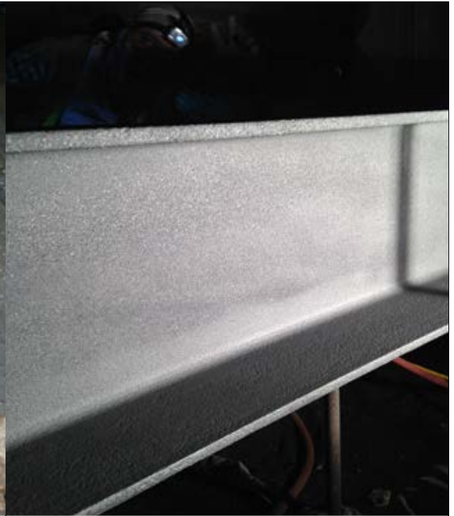
Support beam for Water main after blasting at span C
