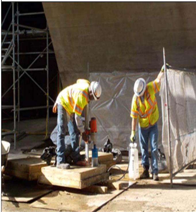
Coring Test Panel for Shotcrete compressive strength specimen
