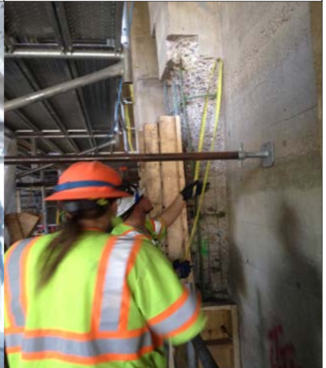
Setting up forms for concrete repair at North abutment
