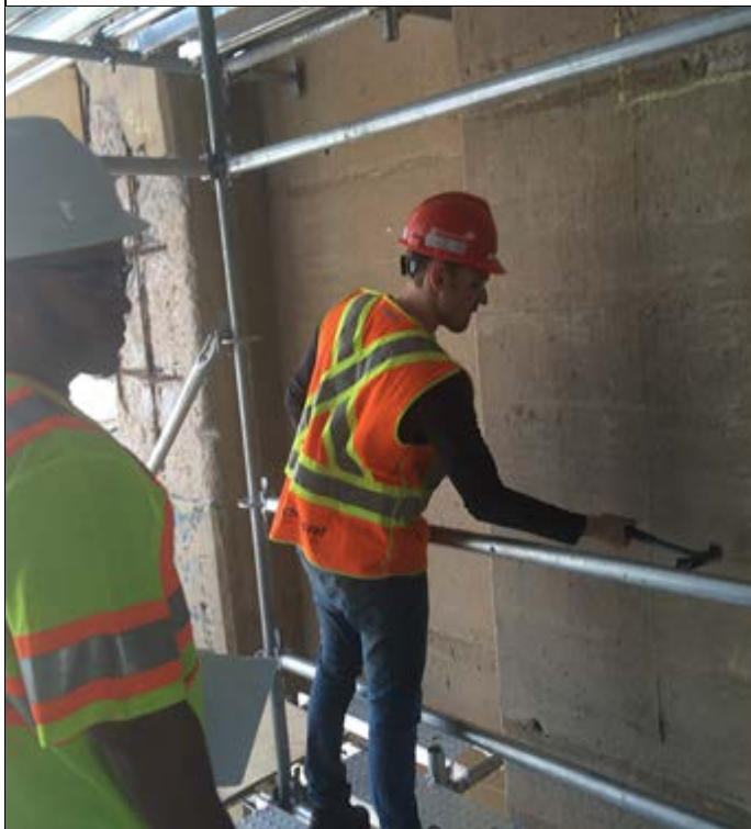
Concrete demolition at North abutment
