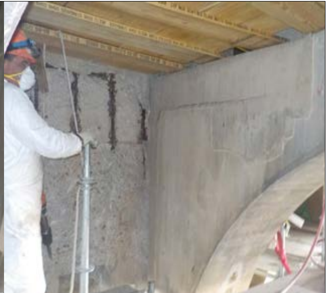
Concrete demolition at North abutment
