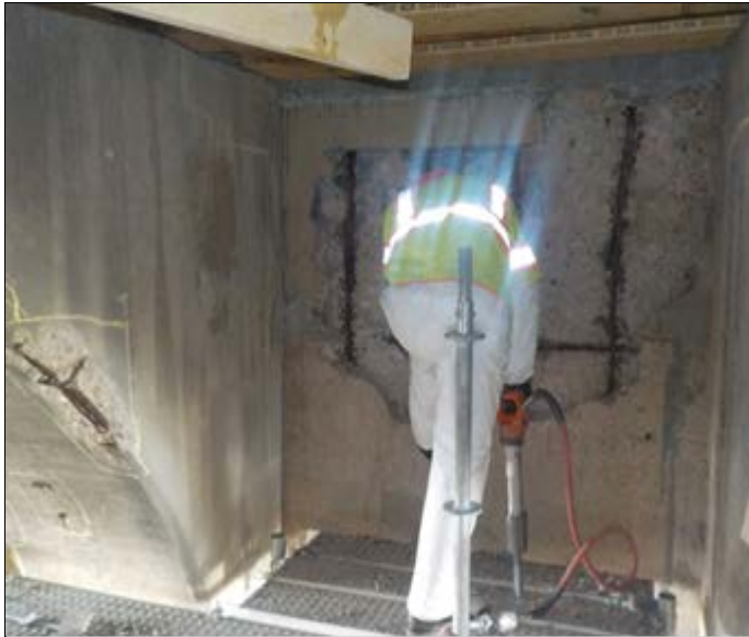
Concrete demolition at North abutment
