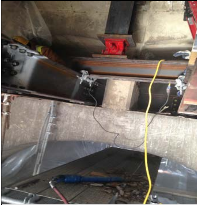
Setup for Repair/Replacement of pedestal at row D column 52.
