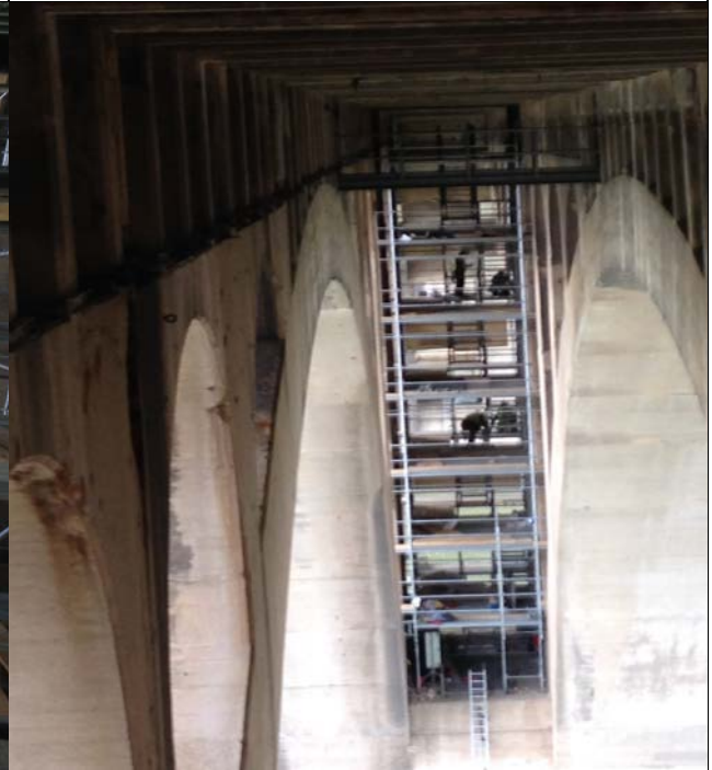
Setup for Repair/Replacement pedestal at row D column 52
