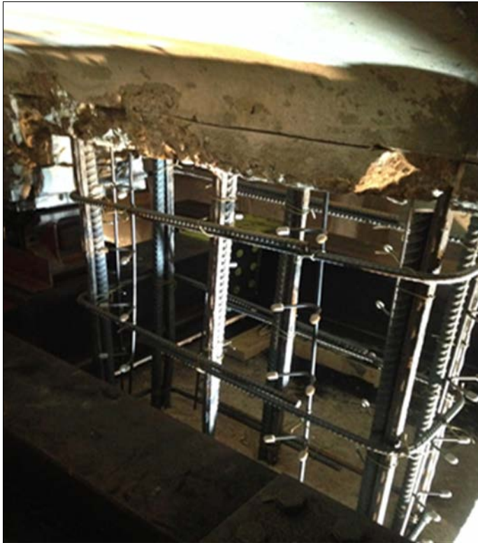
Setup for Repair/Replacement pedestal at row D column 52
