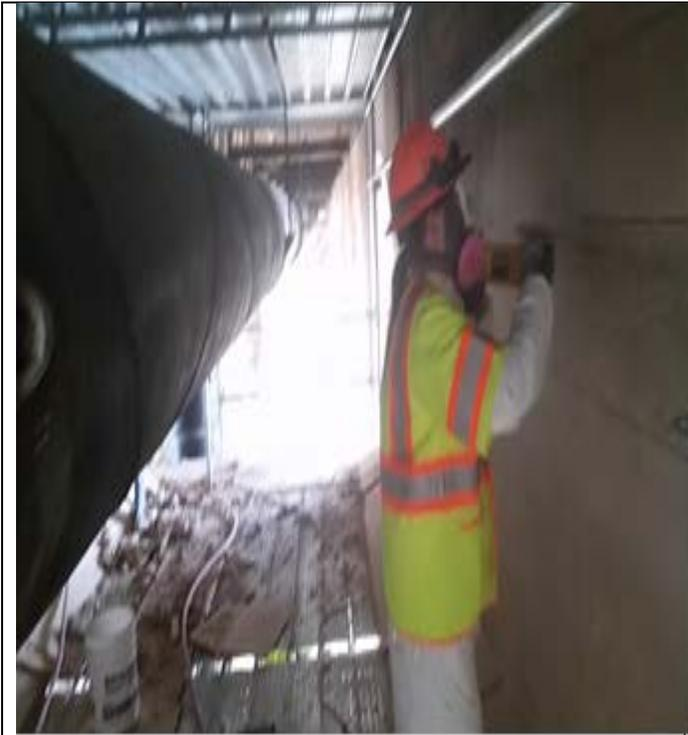
Concrete demolishing and saw-cutting at pier 4
