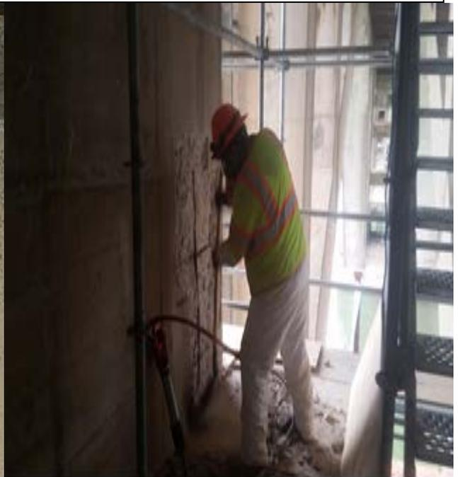
Concrete demolishing and saw-cutting at North abutment
