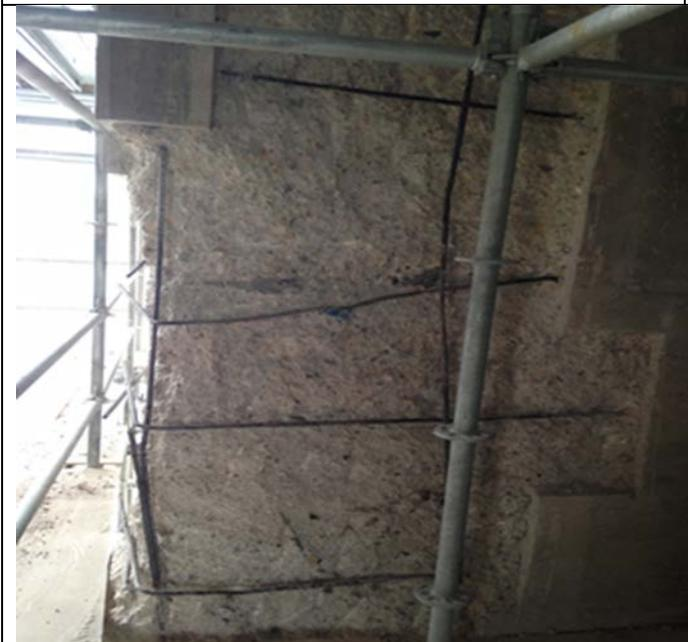
Concrete demolishing and saw-cutting at pier 4
