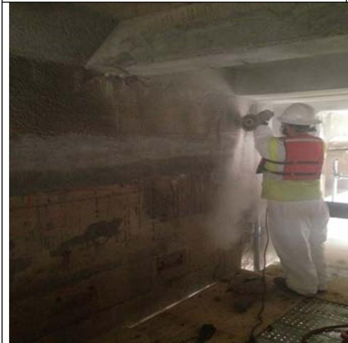
Concrete demolishing and saw-cutting at North abutment
