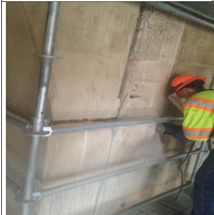
Concrete demolishing and saw-cutting at North abutment
