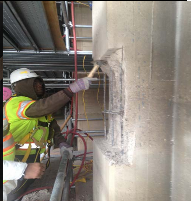
Inspection and sounding at North abutment
