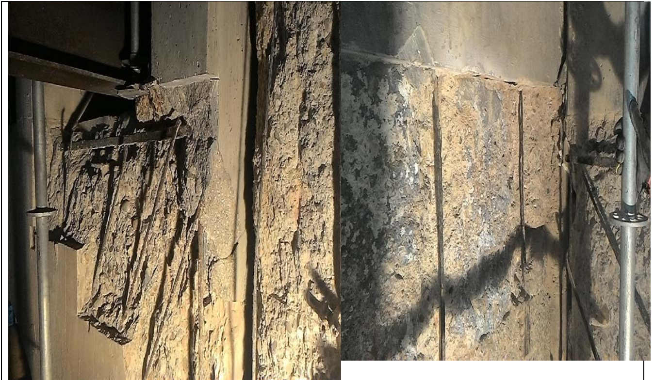
Concrete demolishing at North abutment.
