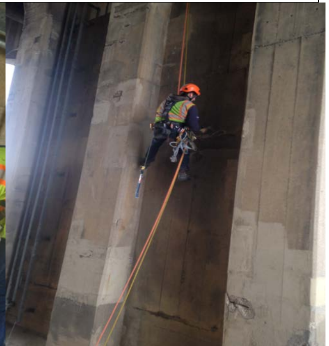
sounding and scaling at the mid arch span C
