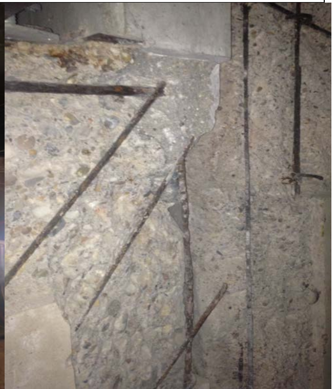
Concrete demolishing at North abutment
