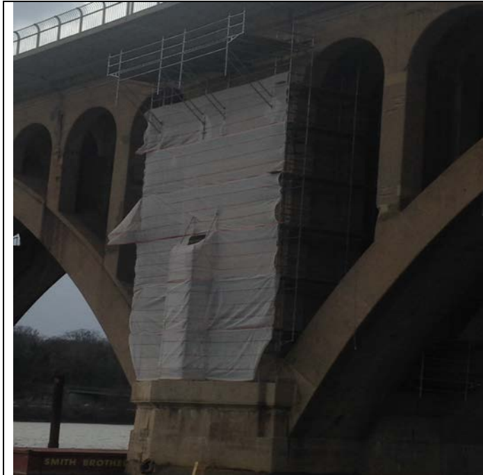
Installing net on Pier 4
