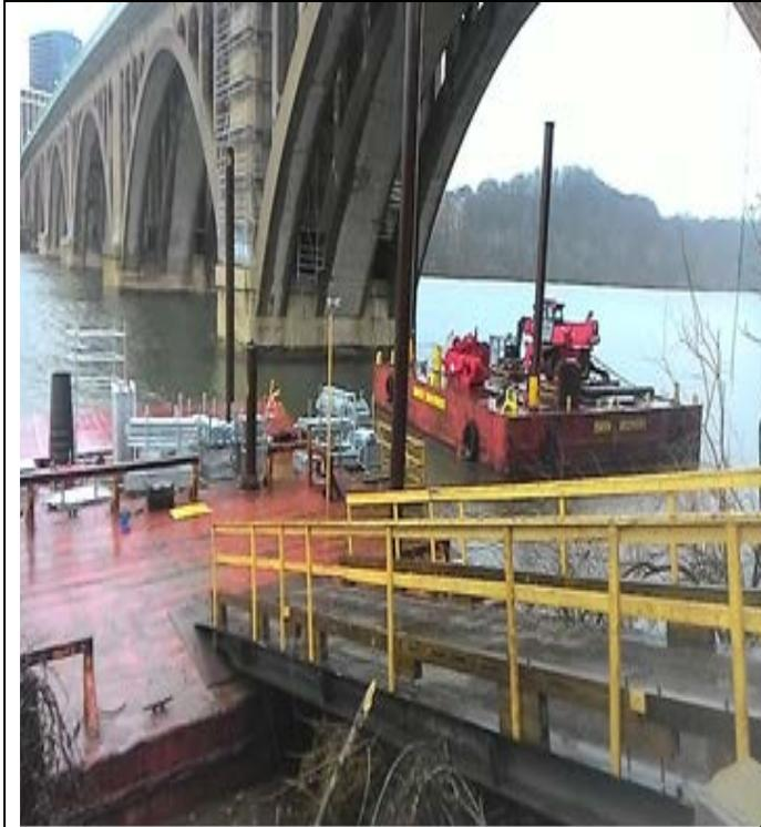
Loading /navigating stockpile of scaffolding to Pier 4
