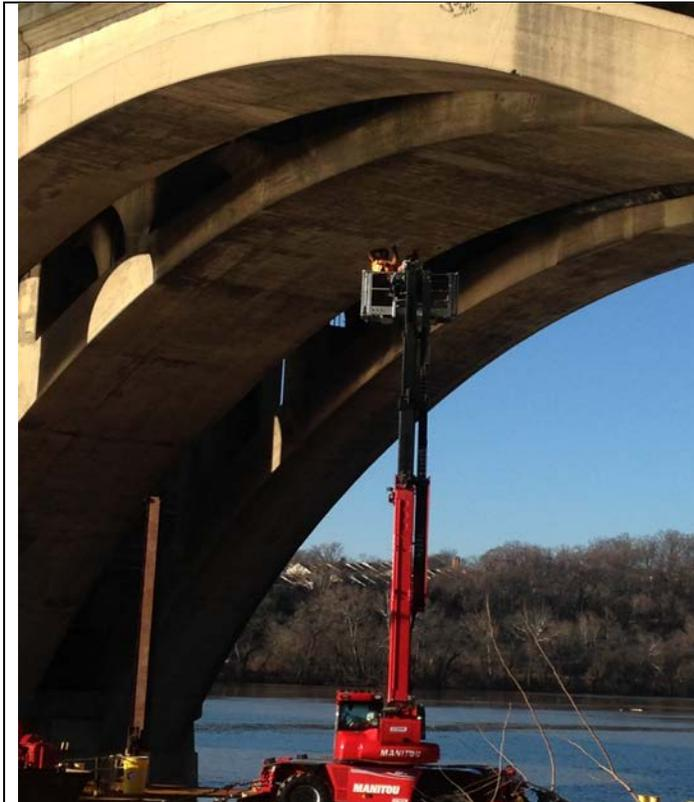
Sounding and concrete scalling at span C
