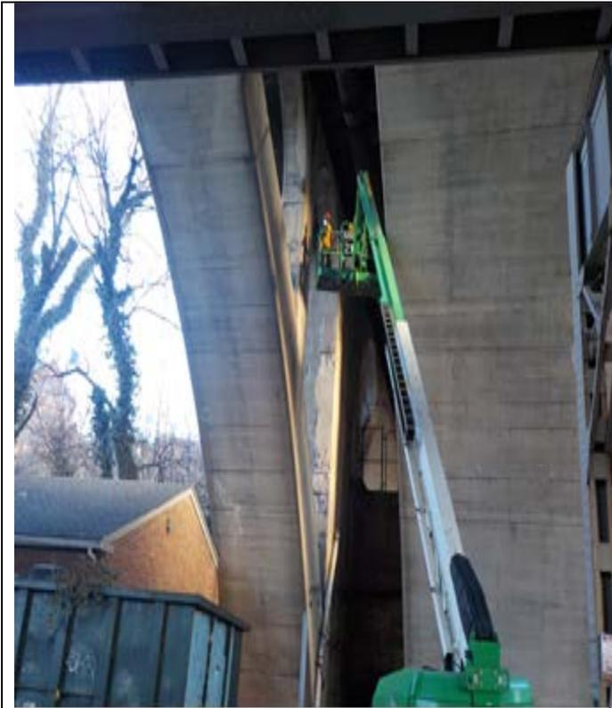
Sounding and concrete scalling at span B
