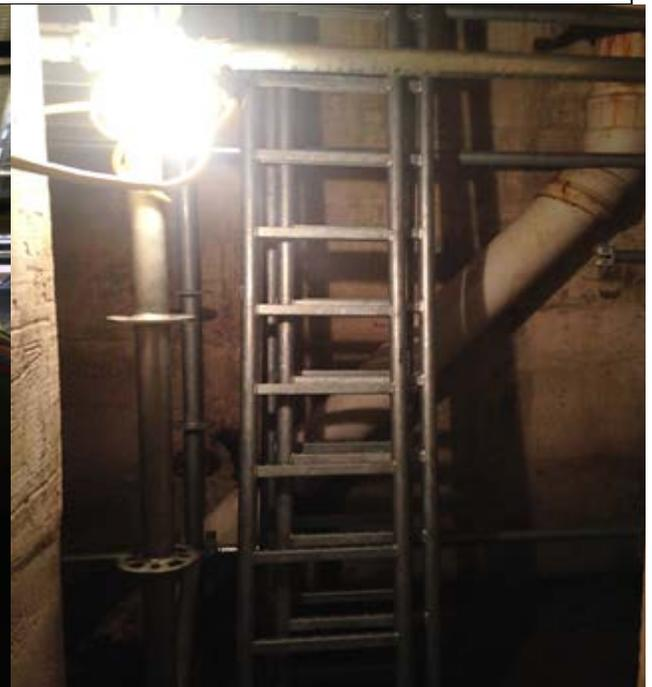
Scaffold and ladders installation inside North abutment chamber
