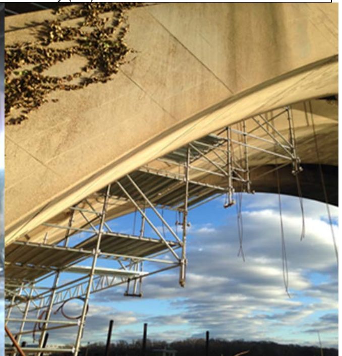
Erecting suspended scaffold from North abutment to pier 4
