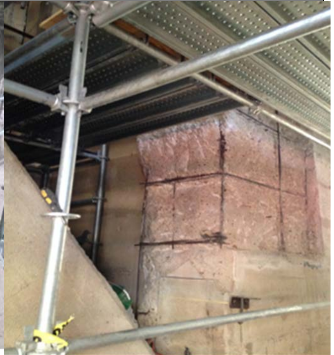
Concrete demolishing at level 1 of bay 5/East pier
