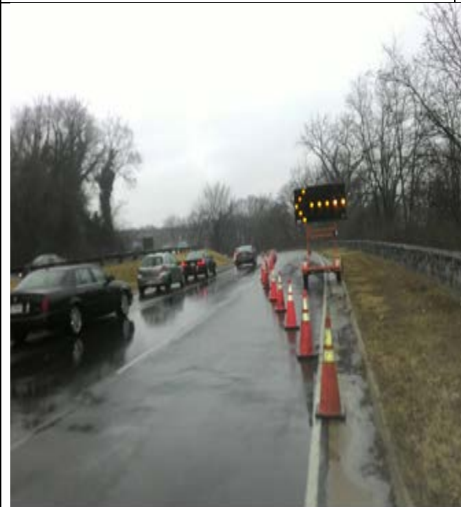
MOT setup on GW Pkwy.( NB) for removing imminent concrete spalls
