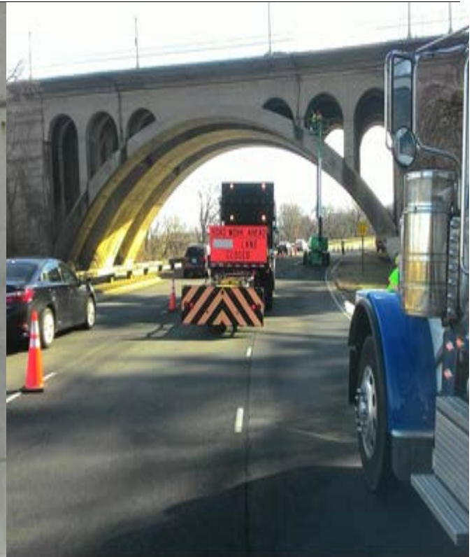
MOT and removing imminent concrete spalls over GW Pkwy (NB)
