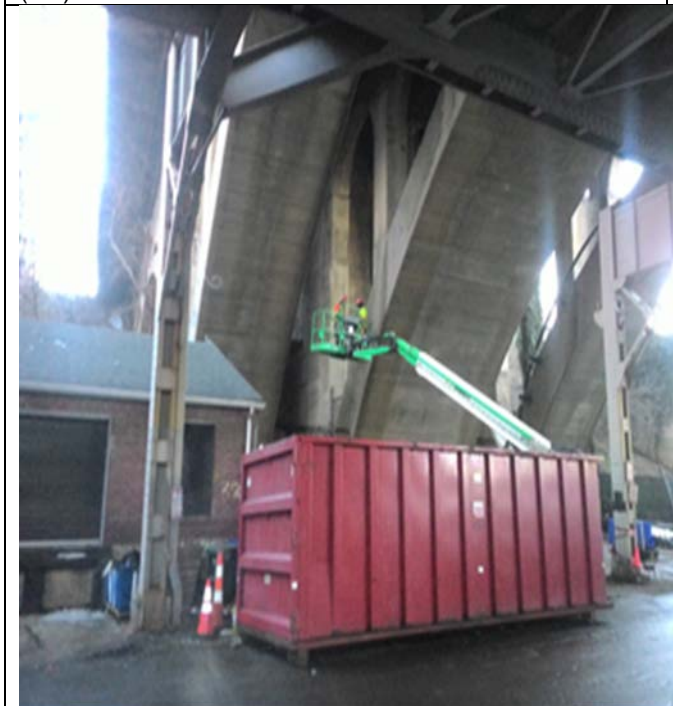
Removing an imminent concrete spall at pier 5 Southside span B
