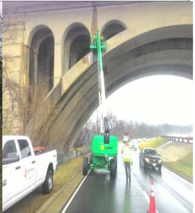
Removing imminent concrete spalls over GW Pkwy (NB)
