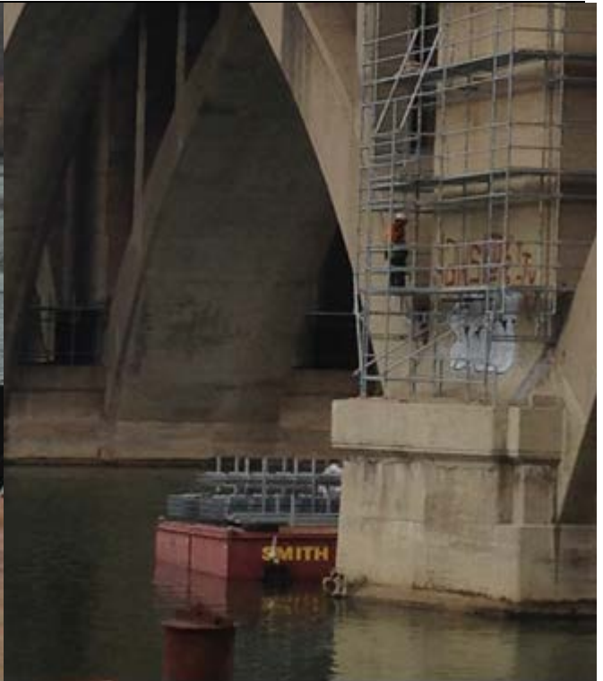
Erecting scaffold system at Pier 4
