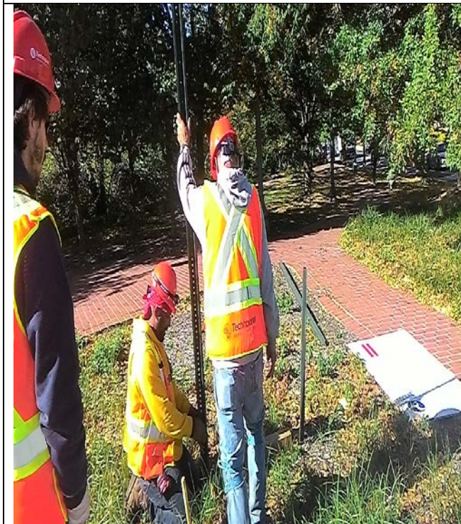
Technopref installing Federal Aid Sign on M Street
