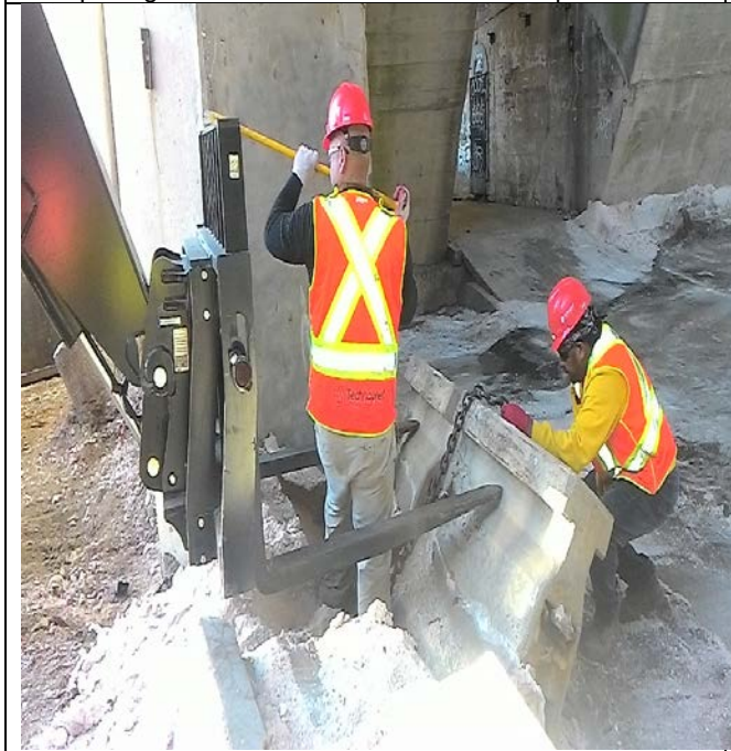
Technopref removing temp PCC barriers around the North abutment NE side
