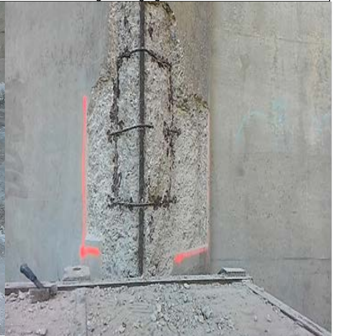
Subcontractor, FIBRWRAP chipped area for mock-up on North abutment east side
