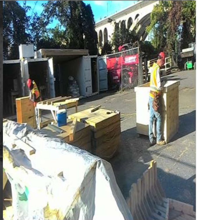
Carpentry work for dock and barges
