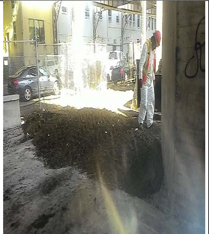
Ramp staging area at North abutment
