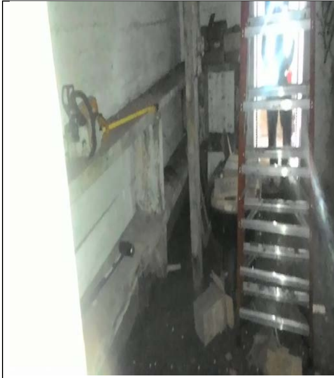
Inside North abutment chamber after cleaning
