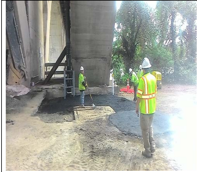
NPL paving over backfill for 2-12 inch main repaired
