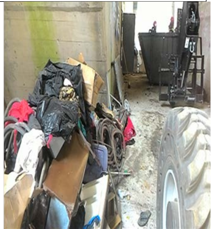
Debris from North abutment chambers
