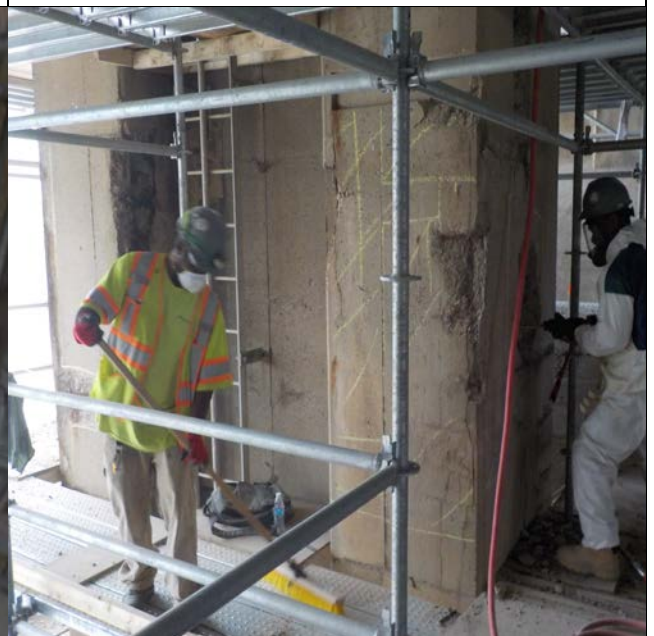
Chipping concrete at Span D
