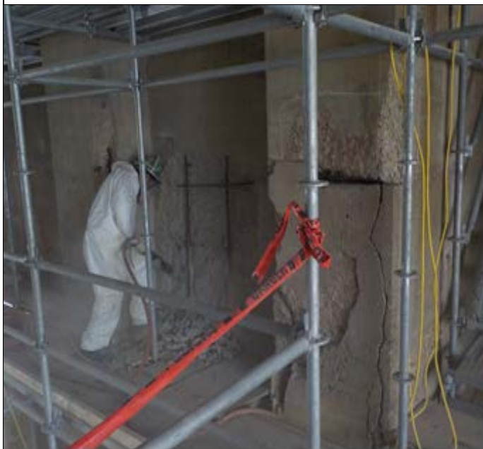
Chipping concrete at Span E
