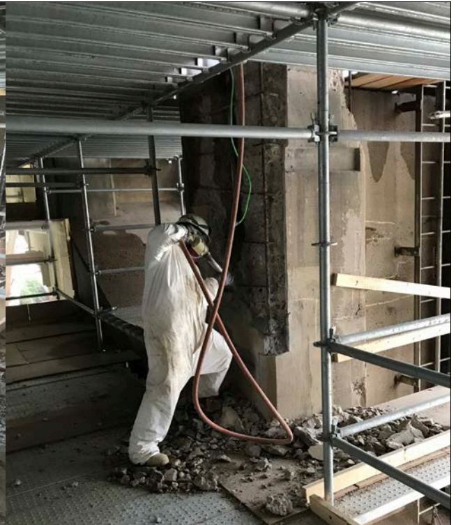
Chipping concrete at Span D
