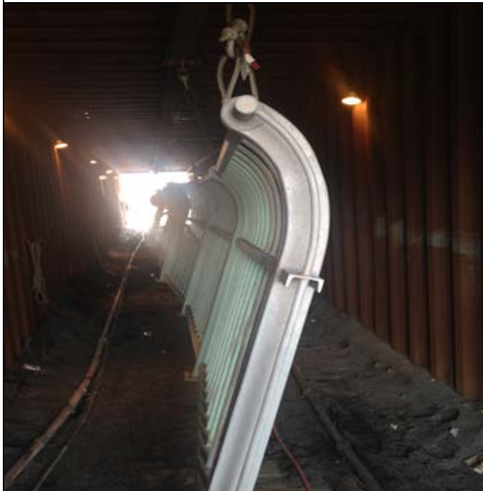
Removing the pedestrian railing and replacing it with temporary railing
