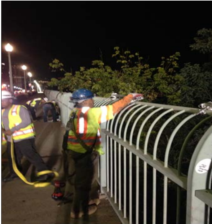
Removing the pedestrian railing and replacing it with temporary railing
