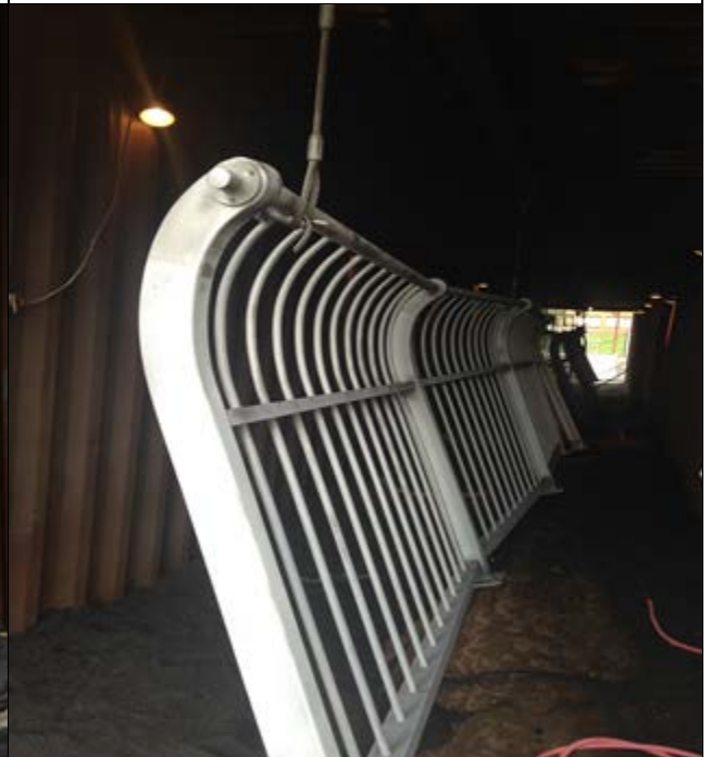
Pedestrian railing preparation before blasting operation at the plant
