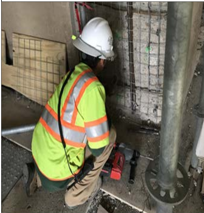
Drilling and installing an anchor for the wire mesh at Pier 4
